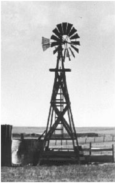
Figure 5. A steel-bladed water pumping windmill in the American Midwest (late 1800's)
