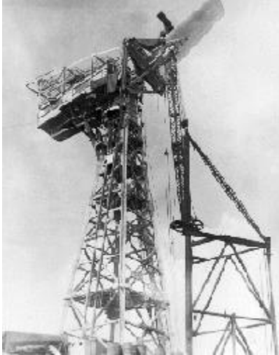
Figure 8. Palmer Putnam's 1.25-megawatt wind turbine was one of the engineering marvels of the late 1930's, but the jump in scale was too great for available materials.
