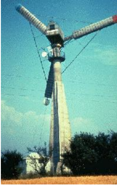
Figure 9. Yes, that's an airframe holding together the three blades of the "Gedser Mølle." Fiberglass later eliminated this design requirement.
