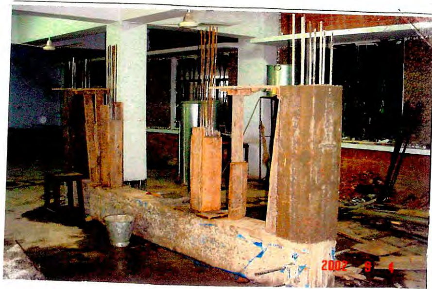
Fig.: 3.4 Construction of the test rig - casting of column in progress.
