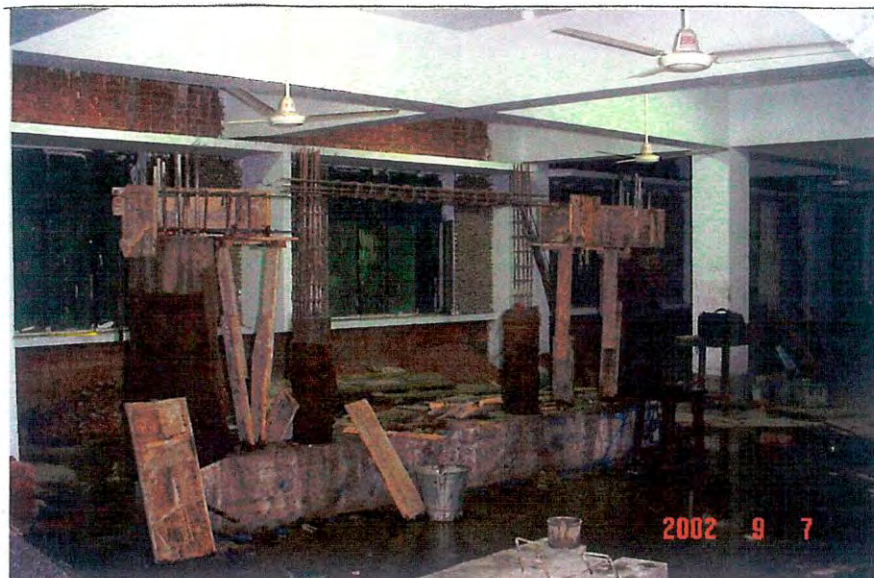
Fig.: 3.11 Construction of the test rig-reinforcement arrangement of the beams.
