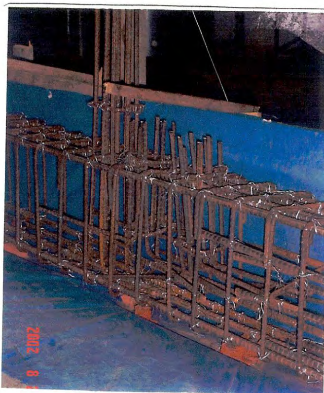
Fig.: 3.3 Close-up view of base reinforcement.
