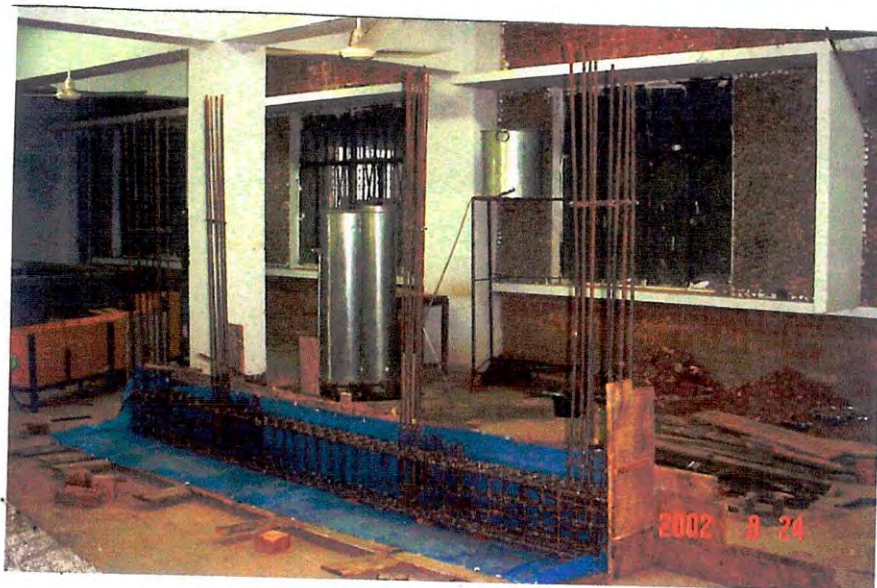
Fig.: 3.2 Construction of the reaction frame - before casting.
