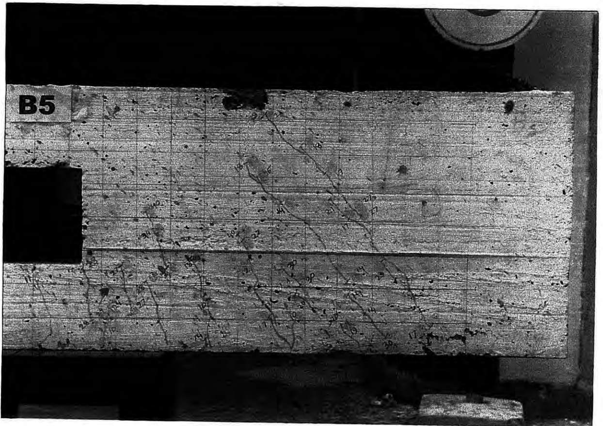
Figure 5.4e Crack pattern of beam B5
