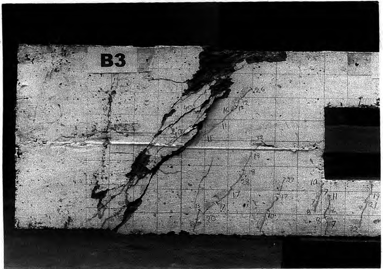
Figure 5.4c Crack pattern of beam B3
