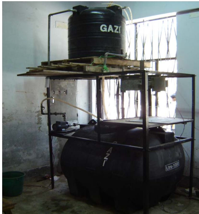
Figure-3.3: Laboratory Raw Water Feeding Arrangement to MSFs
