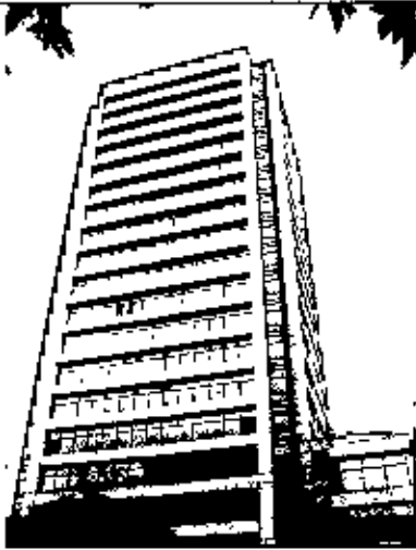
Figure 5.3(a): View of building H03.
