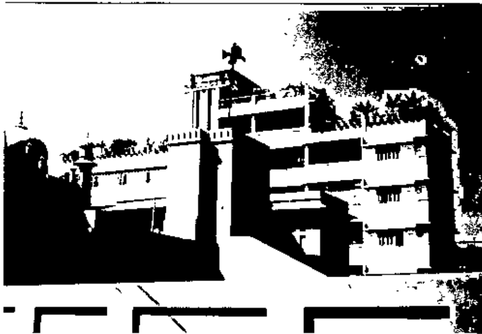
Fig. 5.43 Over imposing six storied structure disturbing the mosque's vicinity.
