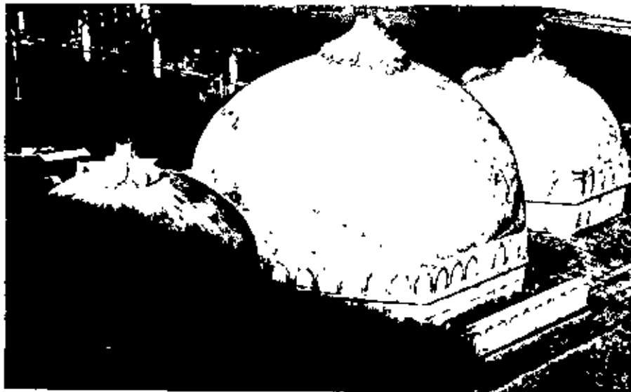
Octagonal base of the dome with merlon pattern-Abmer mosque of Mughal period
