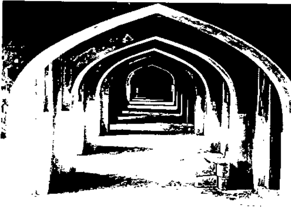
Fig 5.42 The corridor connecting the cell like chambers beneath the podium
