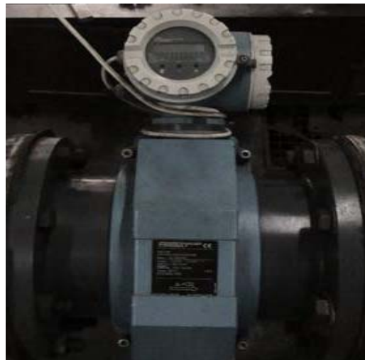
Photograph 4.3: Electromagnetic flow meter.
