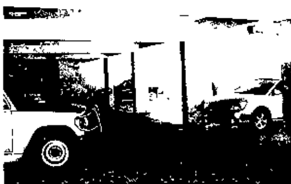
Figure 4.16 Free space for parking in ground level of spot -02, Dhanmondi
