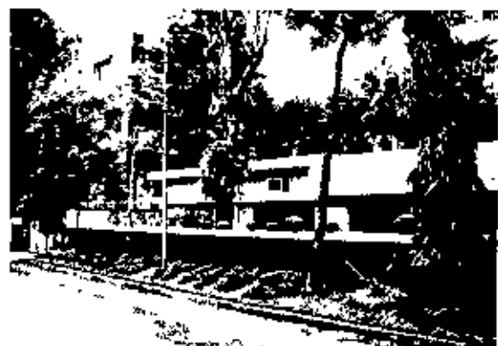
Figure 4.29 Single storied residence on the south of spot -04 in Banani
