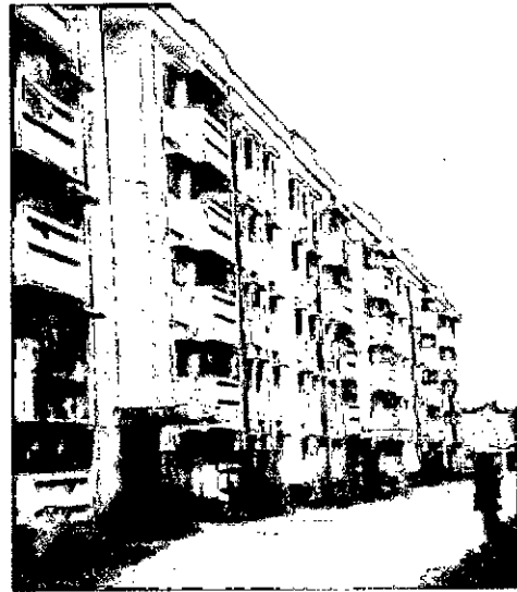
Figure 5.26: New Building in zone D
