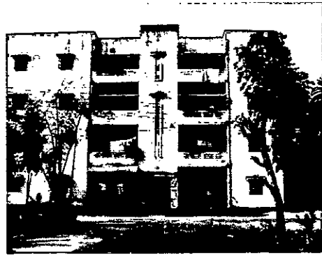
Figure 5.64: Absence of pedestrian walkway
