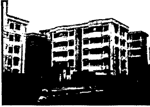
Figure 5.36: New Building in Region G
