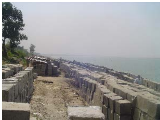
Figure 2.3 : Concrete blocks used in revetment
