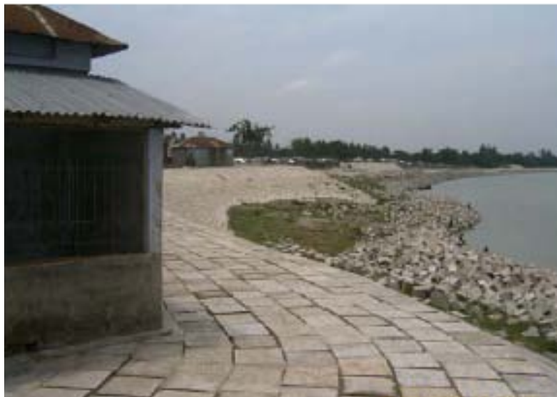
Figure 5.3: Debdanga Revetment along the Right Bank of Jamuna River
