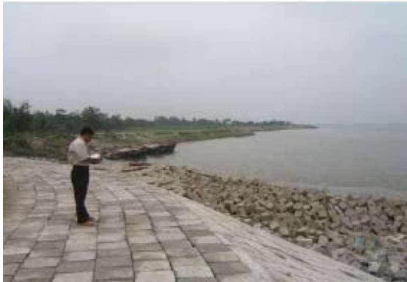
Figure 5.2: Titporol Revetment along the Right Bank of Jamuna River
