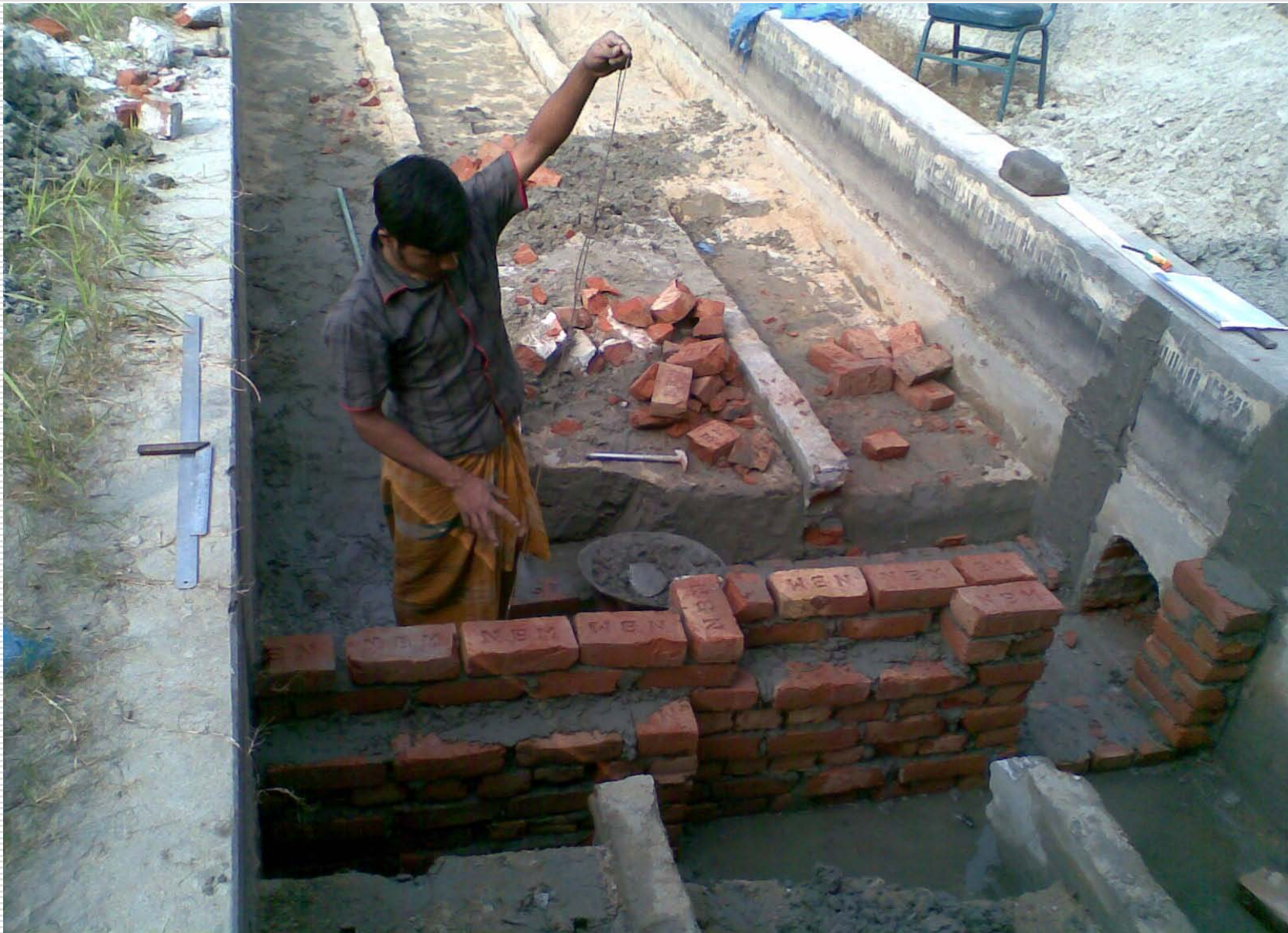
Figure : Construction of diversion chamber
