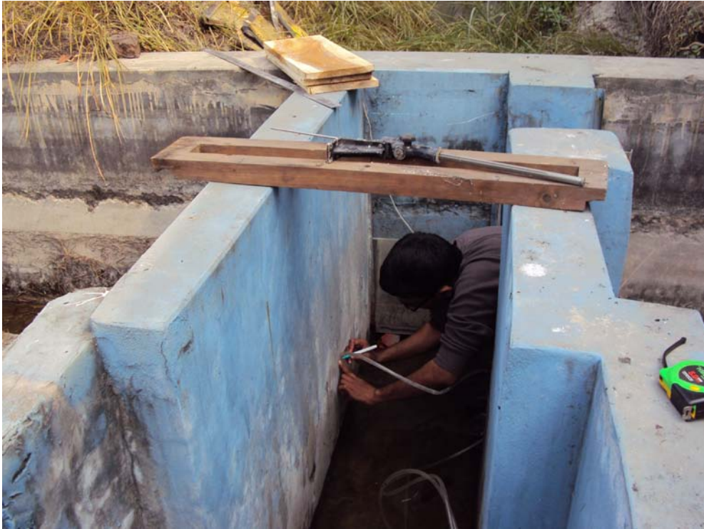
Photograph 4.18: Measurement of the overflow gate height with a level pipe.
