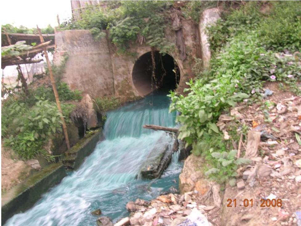
Photograph 3.7: Greenish colored industrial wastewater being discharged near into the Hatirjheel (near Rampura bridge) through the storm sewer (coming from Badda area, Q9)
