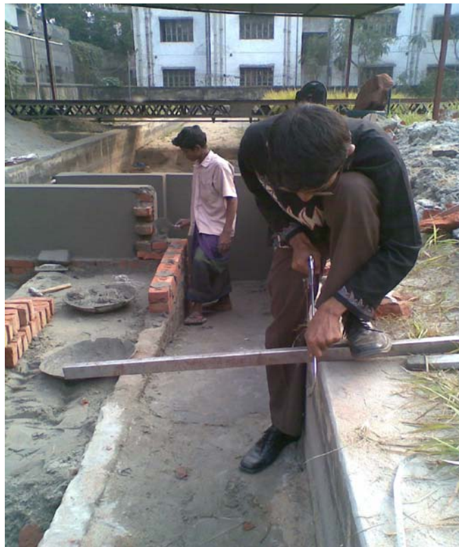
Photograph 4.15: Sliding channel preparation
