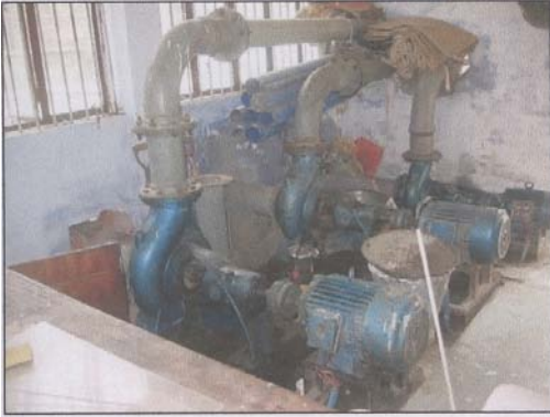
Photograph 4.6: Three centrifugal pumps seen from inside the pump house (I) and the pump outlets (r)
