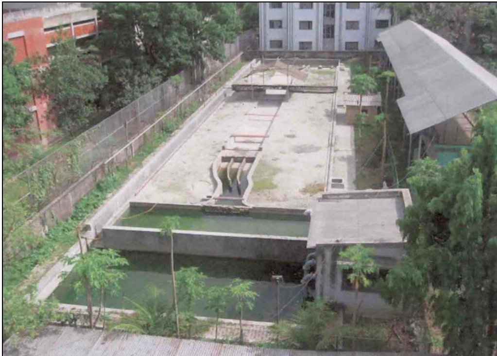
Photograph 4.1: Overview physical model facility
