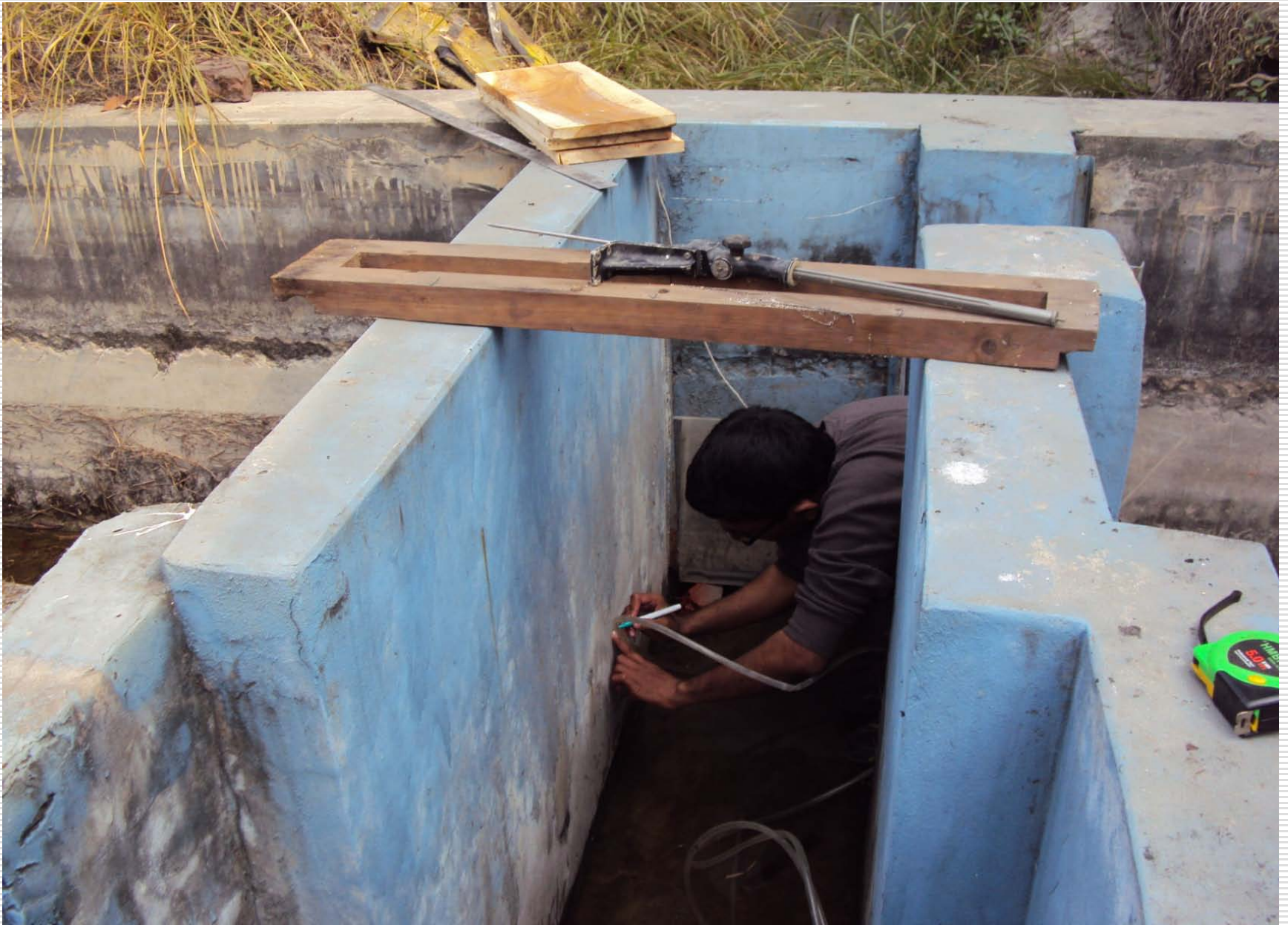
Figure : Measurement of the overflow gate height with a level pipe
