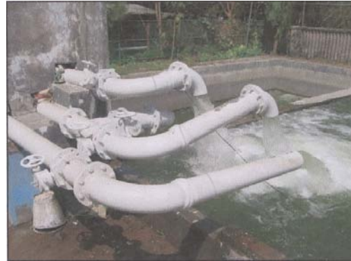
Photograph 4.6: Three centrifugal pumps seen from inside the pump house (I) and the pump outlets (r)
