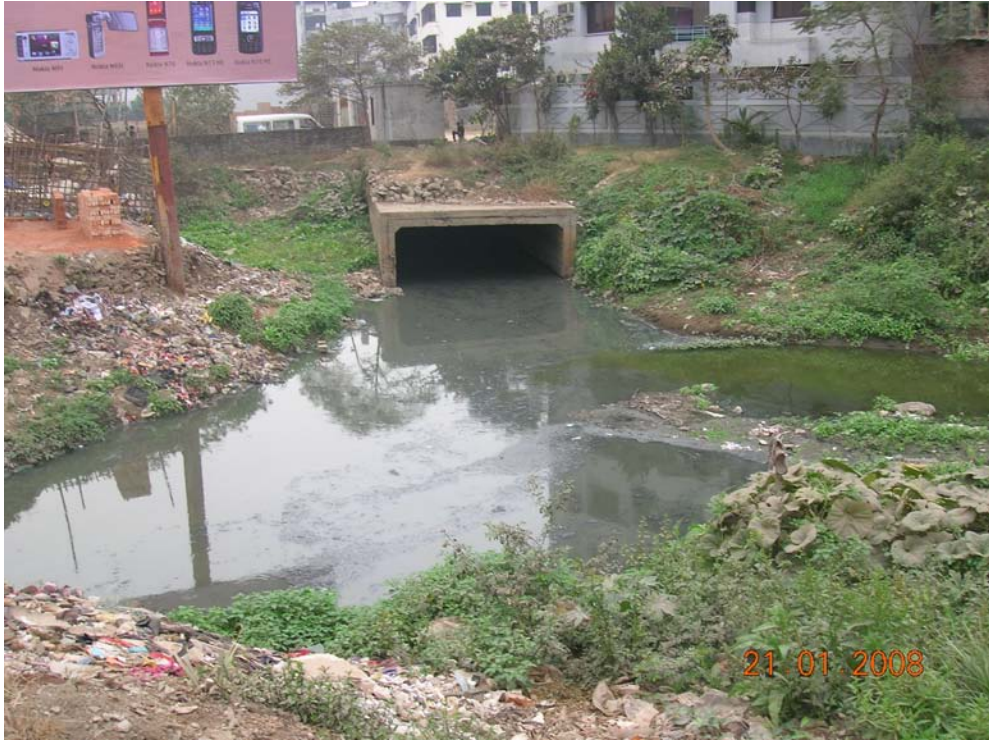
Photograph 3.5: A view of the box-culvert storm sewer at Niketon; flow from the Banani Lake is coming from the right and mixing with the storm sewer discharge (Q6)
