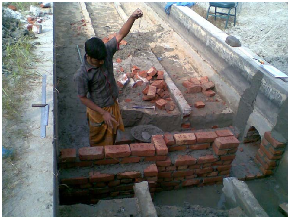
Photograph 4.13: Construction of diversion chamber
