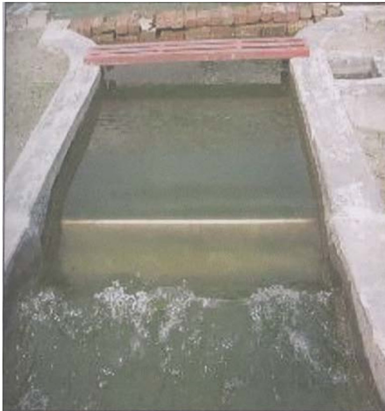
Photograph 4.10: Rehbock weirs at the start point of the flume
