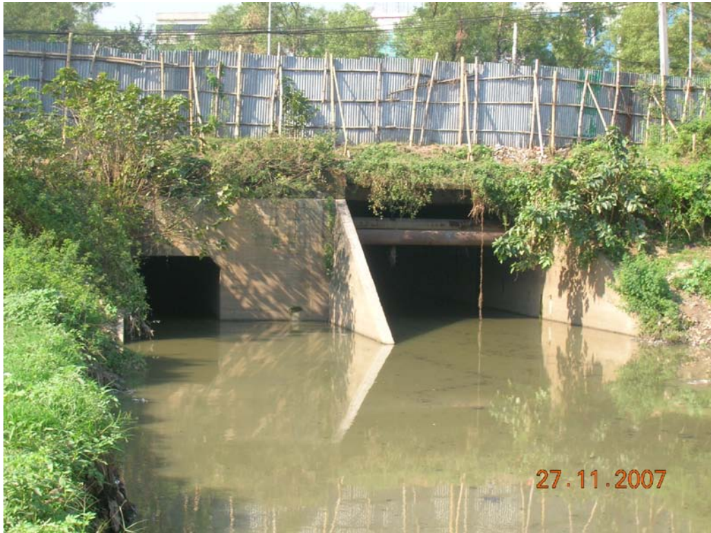
Photograph 3.1: Storm sewer outfall behind Sonargaon Hotel (Q1)
