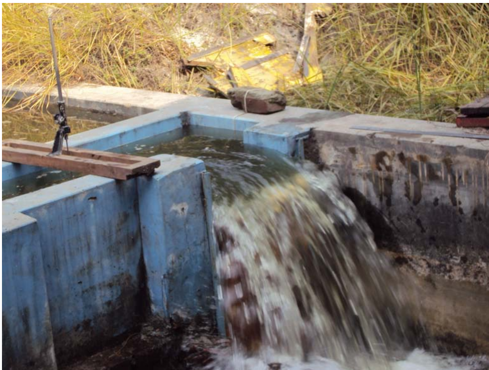
Photograph 4.25: Model is running highest gate height and high discharge. (discharge= 0.109 \text{ m}^3/\text{s} and gate height=692mm)
