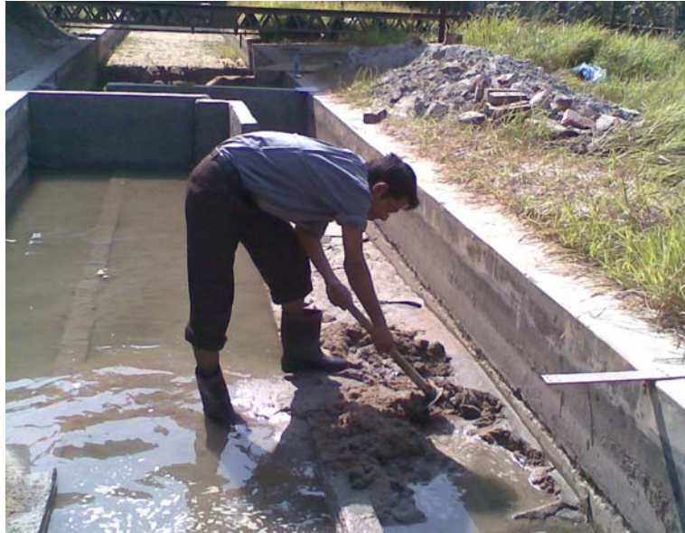
Photograph 4.16: Removing bed sediment from channel
