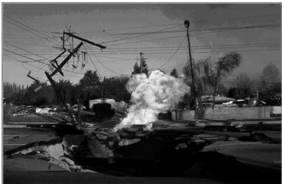
Figure 2.6: Burning Gas Main Ruptured by Lateral Movement, Balboa Blvd in Granada Hills, 1994 Northridge Earthquake
