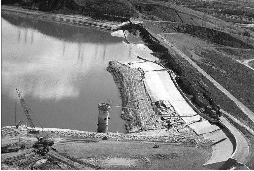
Figure 2.8: Lower San Fernando Dam Suffered an Underwater Slide during the San Fernando Earthquake, 1971
