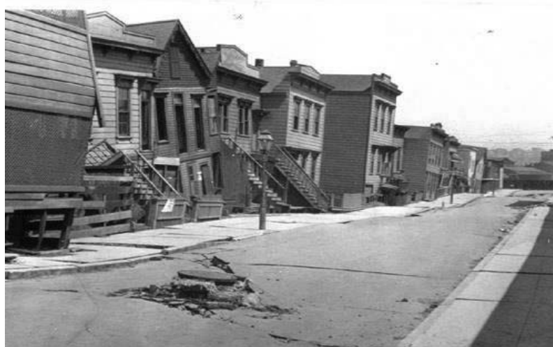
Figure 2.11: Settlement and Disruption of Ground and Pavement over Filled Ground, Dore Street, 1906 San Francisco Earthquake
