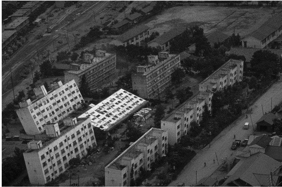
Figure 2.5: Collapse/Damage of Buildings during 1964 Niigata Earthquake
