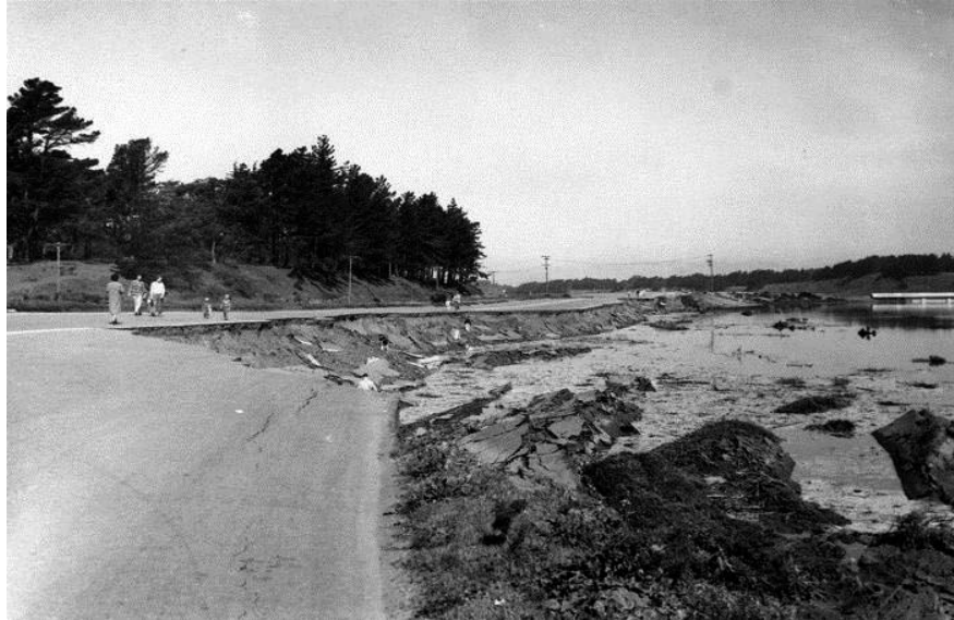
Figure 2.12: A Small Flow Slide along the Shore of Lake Merced in San Francisco in 1957
