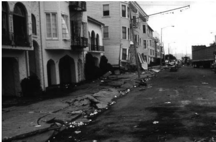
Figure 2.9: Walkway and Pavement Buckled by Ground Oscillation, Marina District of San Francisco, 1989 Loma Prieta Earthquake
