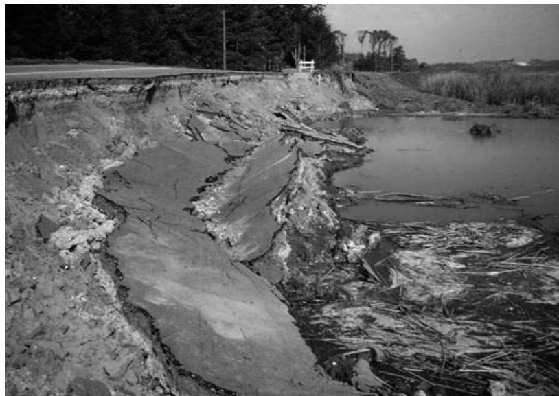
Figure 2.13: Flow Failure in Highway Fill, Lake Merced, 1957 Daly City Earthquake
