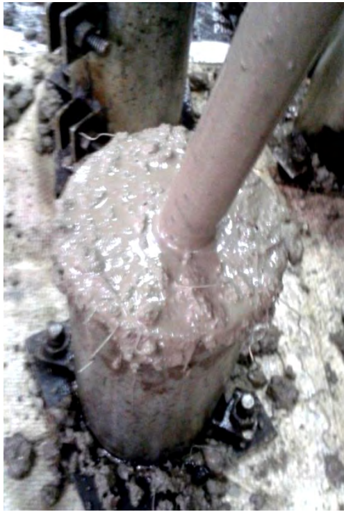
Fig 3.15: Compaction using vibrator machine
