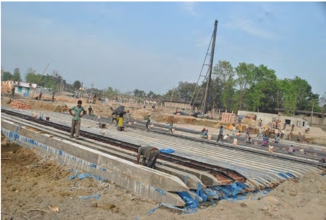
Figure A1 Spliced Precast RC Concrete Piles before driving (Source: PWD)
