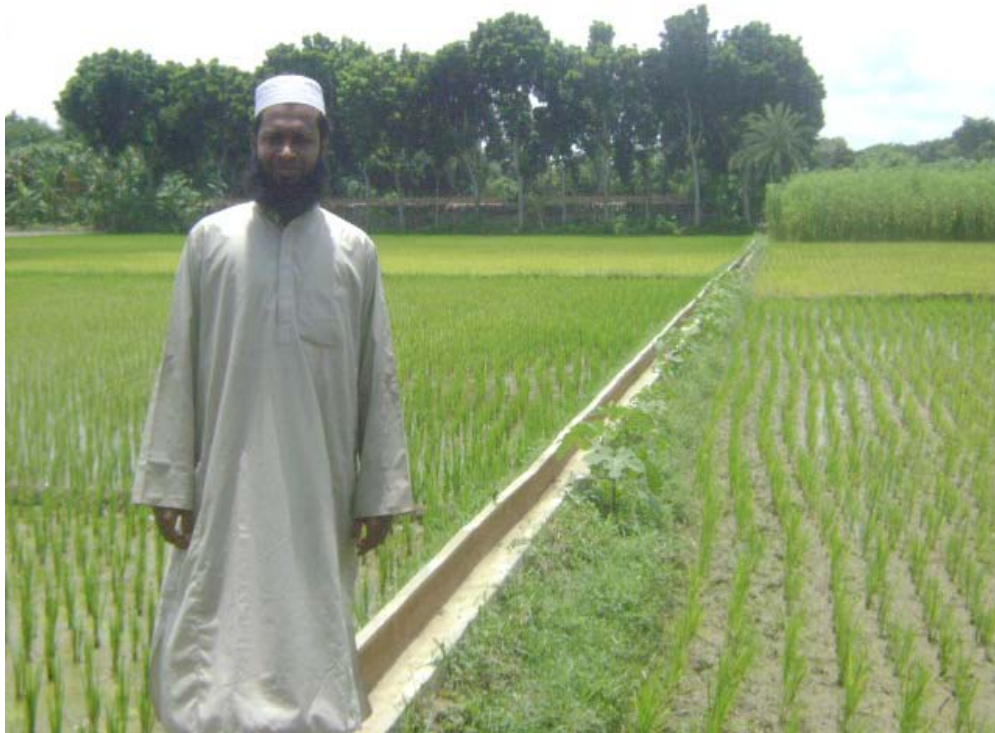
Fig. 3.5: Lined Canal in Haridhali Scheme
