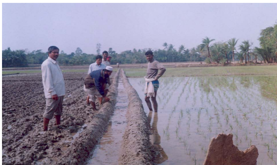
Fig. 3.8 Compacted Earthen Canal in Ganesh More Scheme
