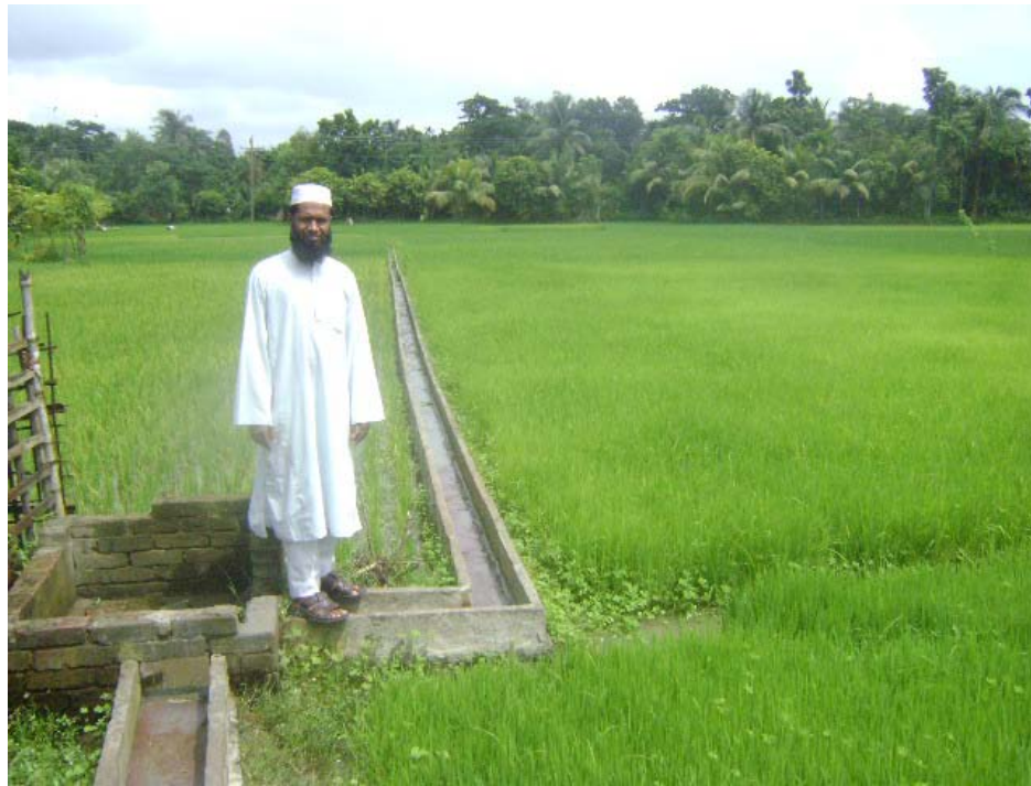
Fig. 3.4: Lined Canal in Agarghata Scheme
