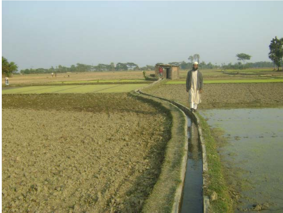
Fig. 3.3: Lined Canal in Ramchandranagar Scheme
