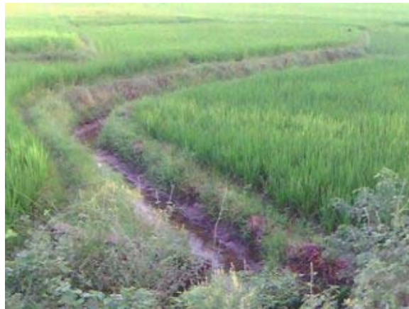
Earthen Branch Canal of Nayagola-Mohananda Irrigation Subproject
