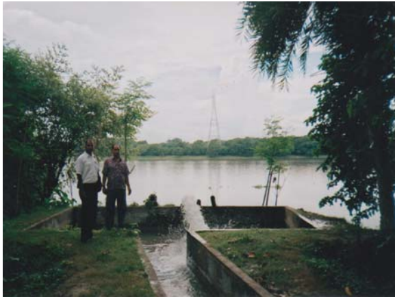
Sump and RCC Canal of Palsha Mahespur Subproject
