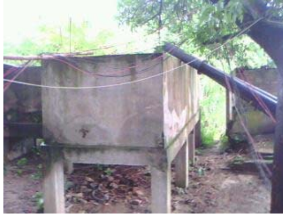
Sump of Nayagola-Mohananda Irrigation Subproject
