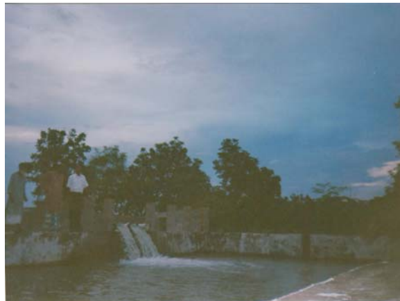
Sump of 2nd lifting arrangement of Mohammadkhani Subproject
