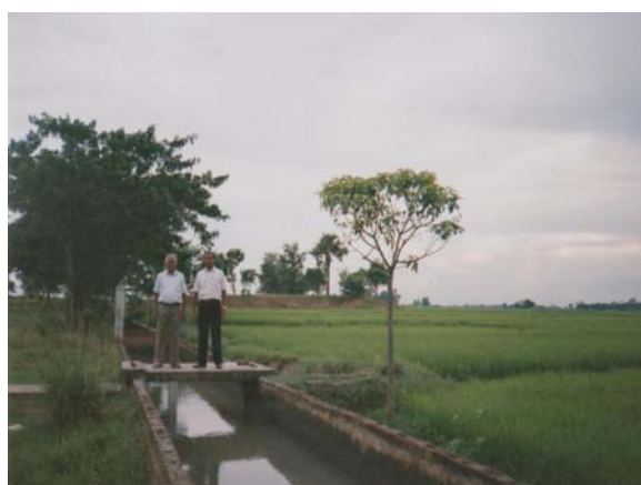
RCC Canal of Mohammadkhani Subproject
