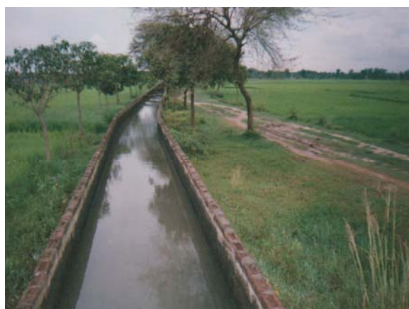
RCC Canal of Mohammadkhani Subproject
