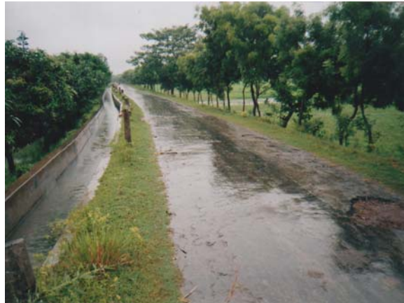
Road Side RCC Canal of Agrani Irrigation CAD Subproject
