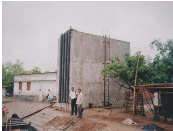
Header Tank of Buried Pipe Irrigation system of Dariapur Subproject
