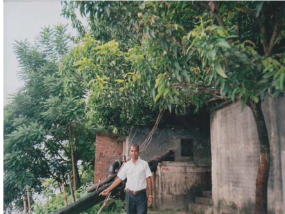
Sump of Agrani Irrigation CAD Subproject
