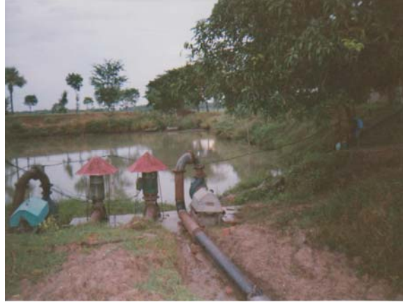
2nd lifting arrangement from pond of Mohammadkhani Subproject
