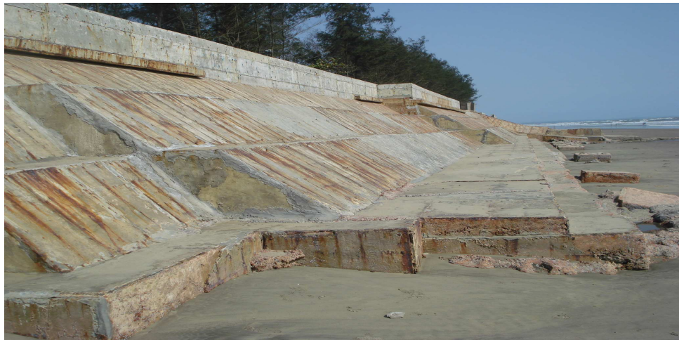
Figure C4: Protection work constructed by Modern Hatchary
