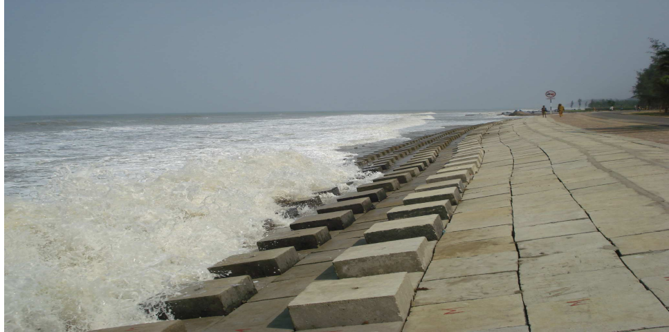
Figure C9: Protection work at Sonarpara, Cox's bazar
