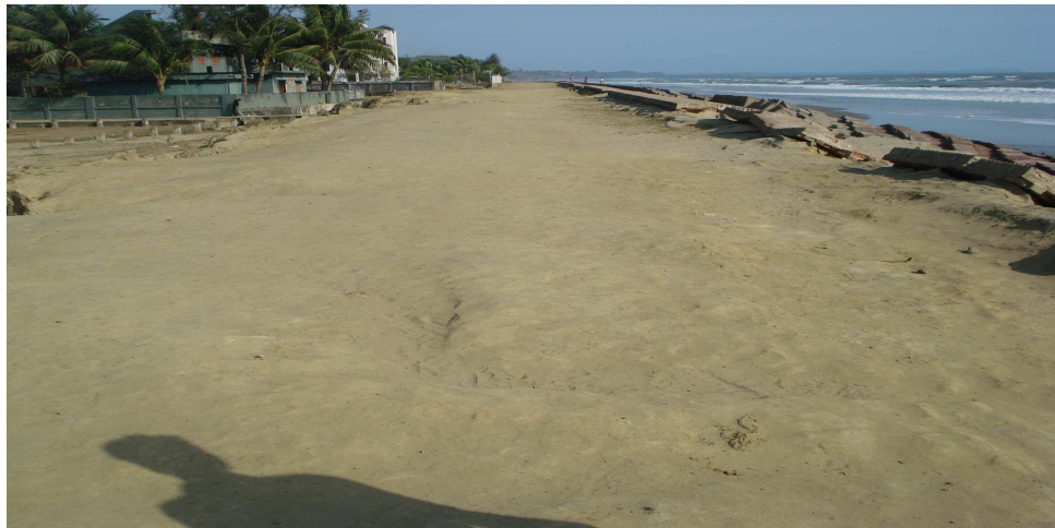
Figure C7: Damaged portion near Brac centre, kalatoly, Cox's bazar
