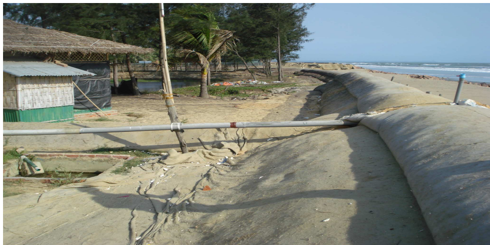
Figure C5: Protection work constructed local businessman
