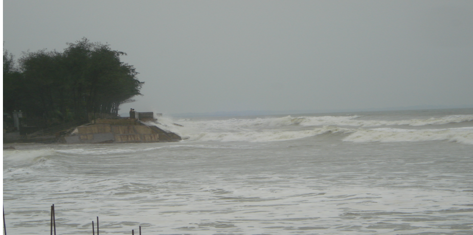
Figure C3: Washed out portion of Marine drive during tidal wave
