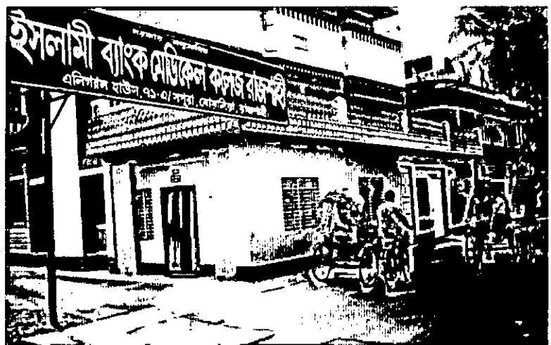
Plate 3: Unauthorized commercial activity in the R/A
