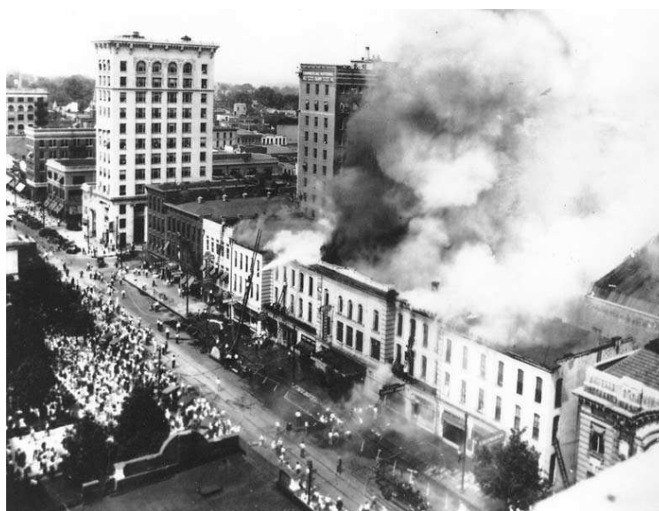
Figure B.5 (b) Hotel Roosevelt fire incident, Florida, December 29, 1963. (Sources: Internet)
