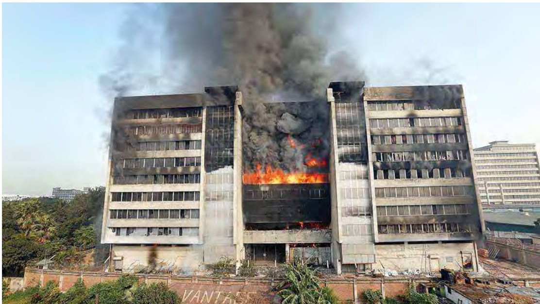
Figure B.1 Fire incident in Standard Garments Ltd., November 24, 2012.
