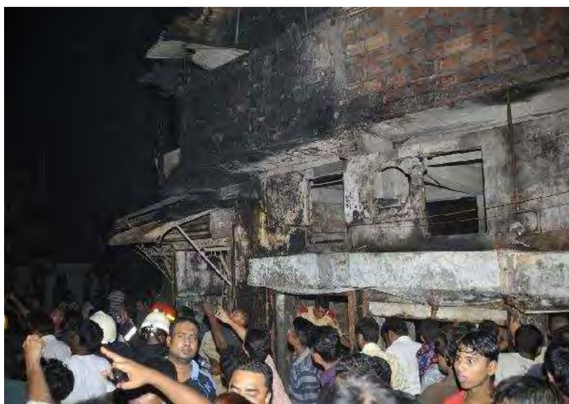
Figure B.3 Fire incident in a chemical factory, Old Dhaka, June 4, 2010.
