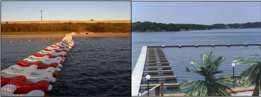
Fig. 1.5 : Floating breakwater
