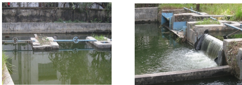
Figure 3.9: Tail gate and flow over tail gate
