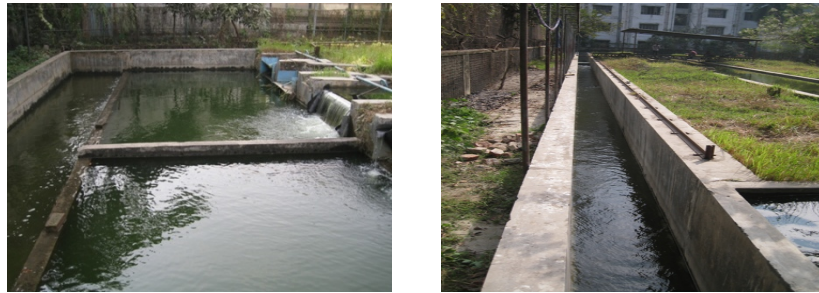
Figure 3.10: Stilling basin and transition flumes
