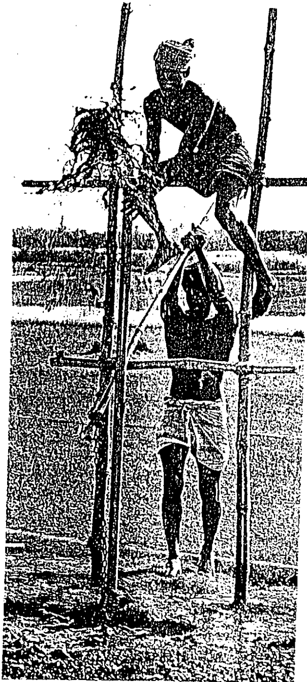
Figure 3.12 Boring Of Shallow Tubewell By Sludger Method
