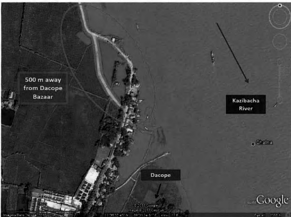
Figure 4-37: Vulnerable Z7606 roadway embankment acting as Berm
