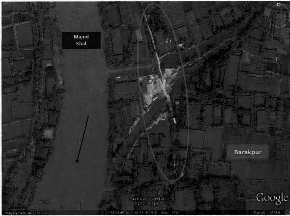
Figure 4-44: Vulnerable area of Z7040 near at Barakpur
