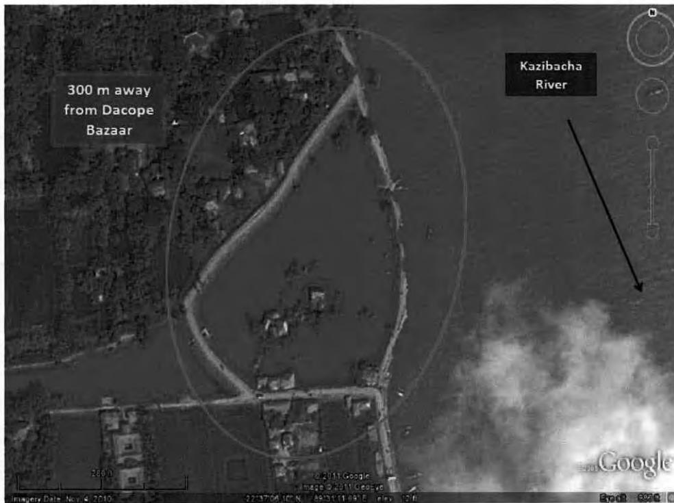
Figure 4-38: Vulnerable location along Z7606 near Dacope Bazar
