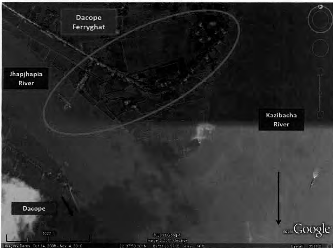
Figure 4-35: Very risky road (Z7606) embankment at Dacope ferry ghat
