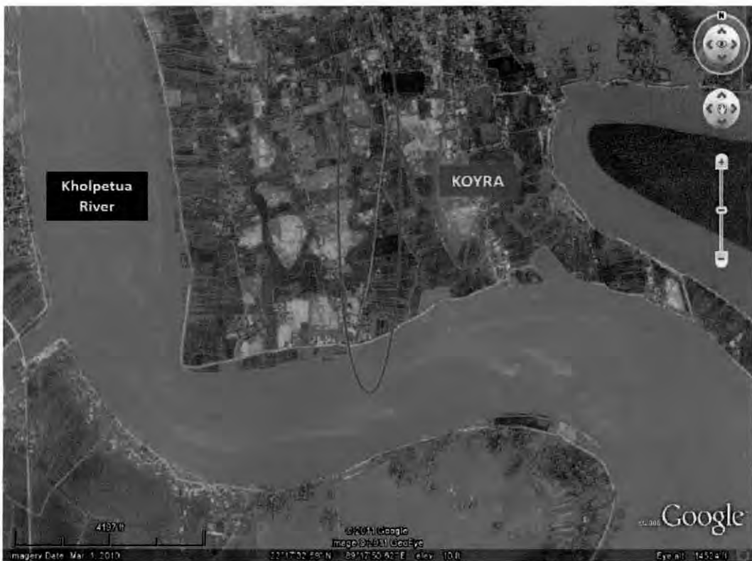
Figure 4-30: Vulnerable areas along Z7604 near Koyra Ferry Ghat
