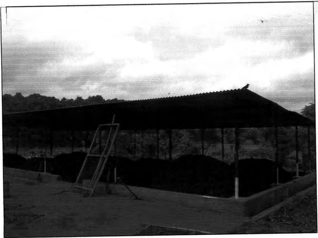
Figure B 7: Aerobic composting plant prepared & maintained by BASA at Gazipur
