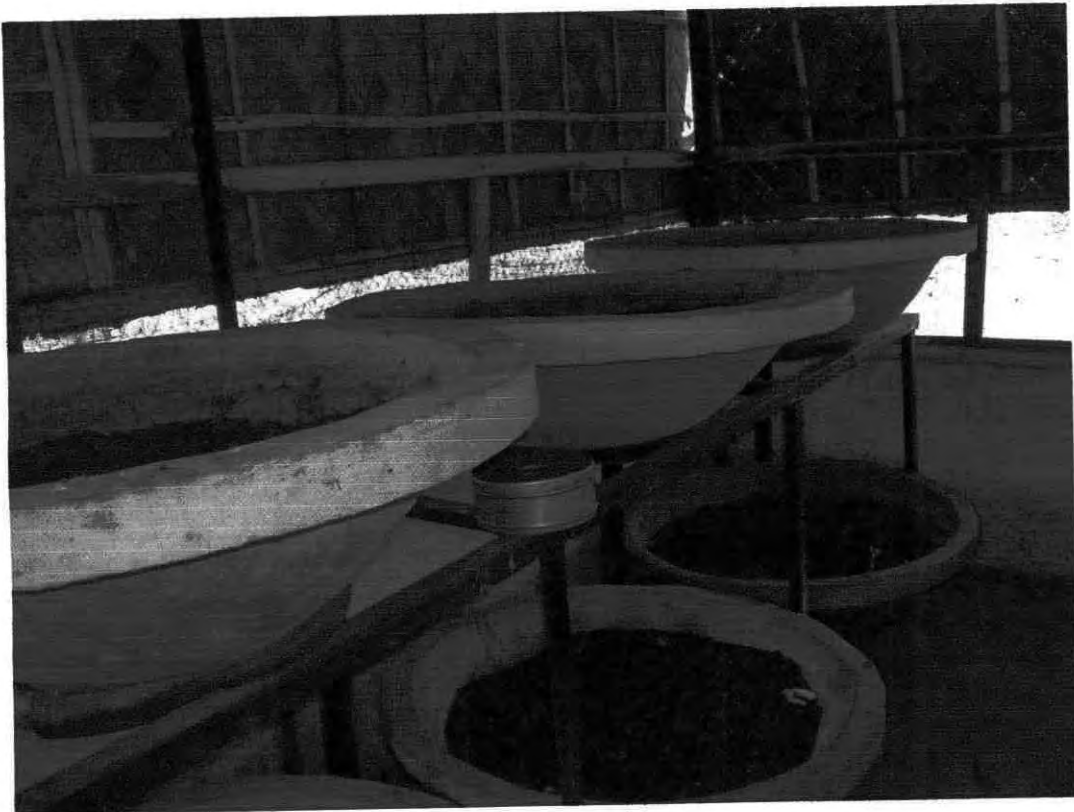
Figure B 6: Vermicomposting plant developed by BASA at Gazipur
