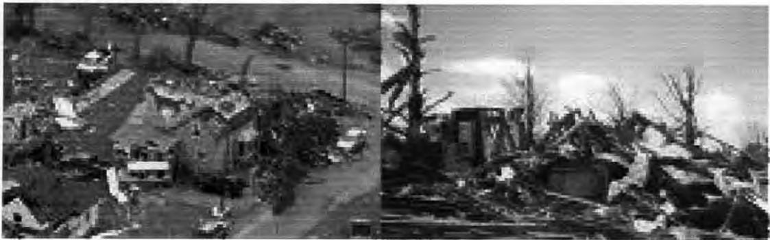
Figure 2.24 Damages occurred by Tornado
