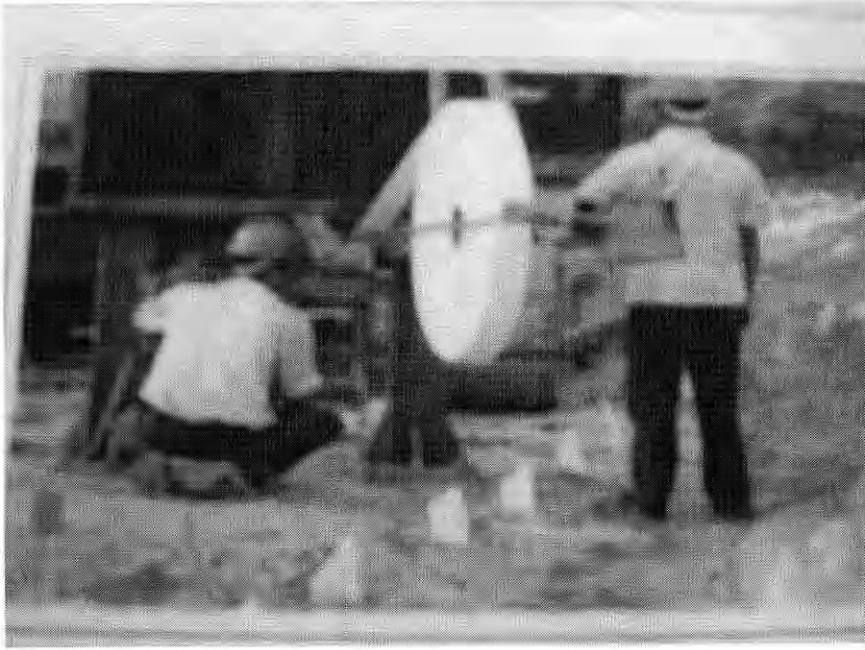
Figure 2.16: Flexi Drain Installation Process in Kaliakoir Bypass
