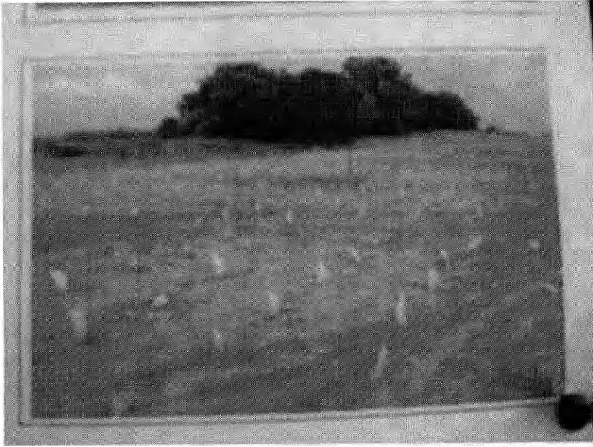
Figure 2.14: Synthetic PVD Used in the Kaliakoir Bypass, Bangladesh
