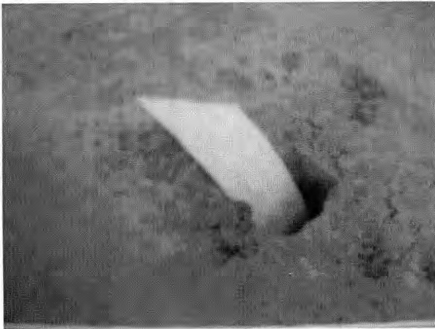
Figure 2.15: Flexi Drain Installation Method in Kaliakoir Bypass
