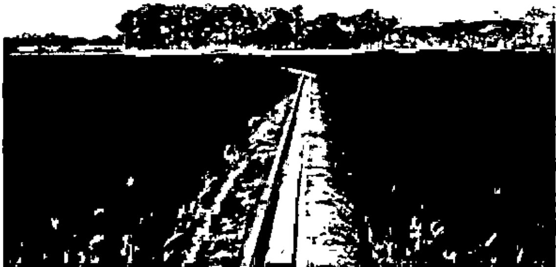
Fig. 3.9. A view of pre-cast canal in Study area.
