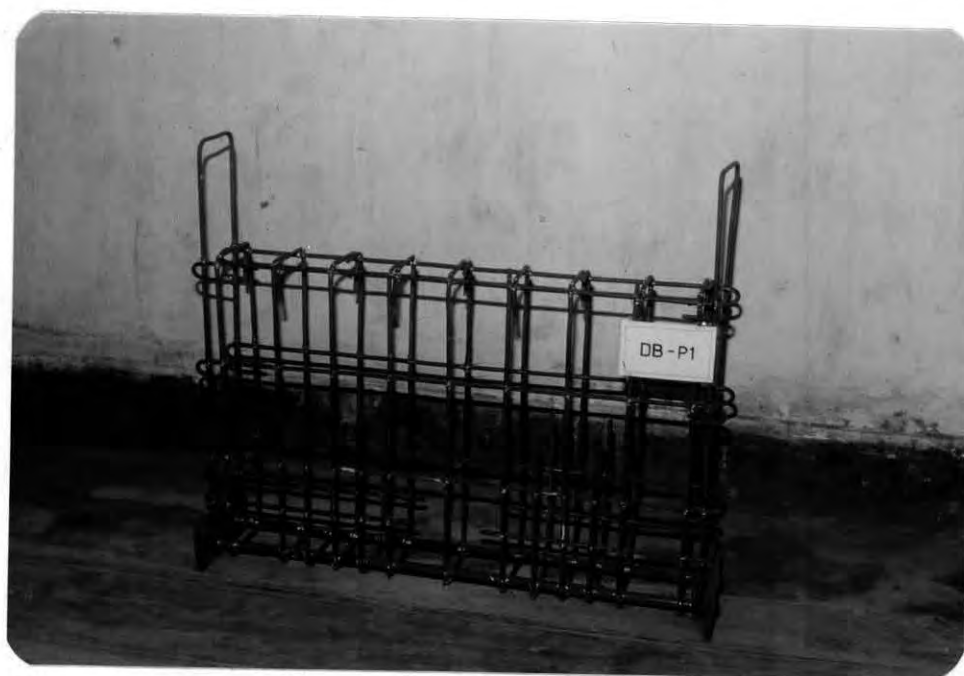
Fig. 4.17 Reinforcement Assembly for Beam DB-P1
