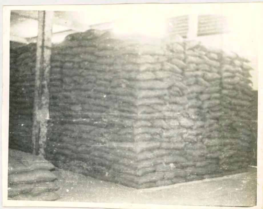
Fig. 4.3 Loading of fertilizer bags closely near to the column.
