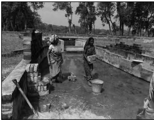
Figure A.7: Carrying of Bricks for Construction
