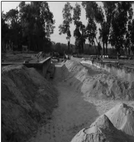
Figure A.3: Placing of Sand at Model Bed
