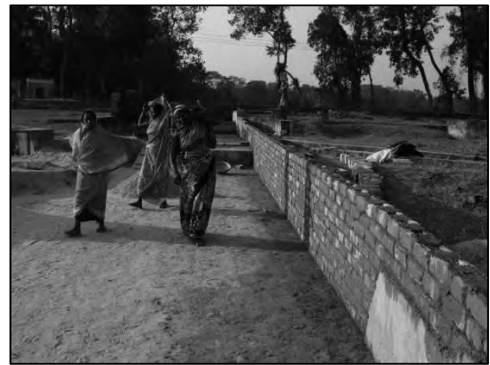
Figure A.8: Construction of MC Boundary
