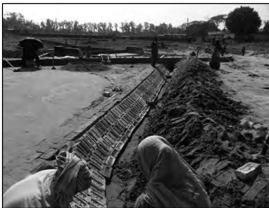
Figure A.15: Construction of Fixed Bed
