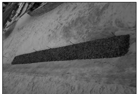
Figure A.46: Launching Apron at Initial Stage (Geo-bag of 738 kg)
