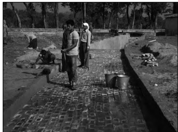
Figure A.16: Brick Flat Soling
