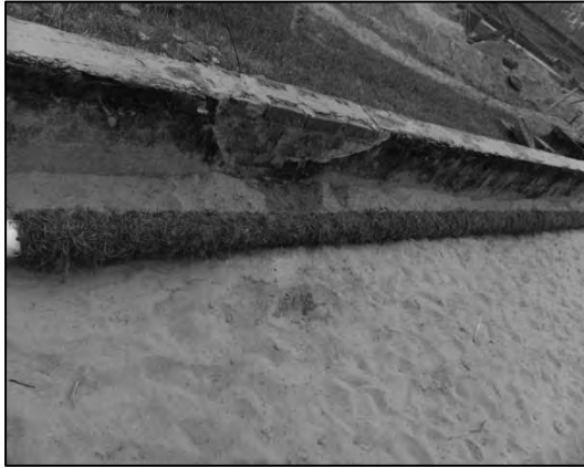
Figure A.11: Rapping of Drainage Pipe with Coconut Fiber
