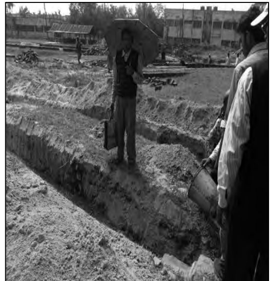
Figure A.4: Layout Fixation for Model Boundary
