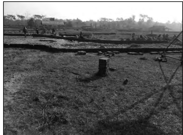
Figure A.22: Bench Mark Fixation
