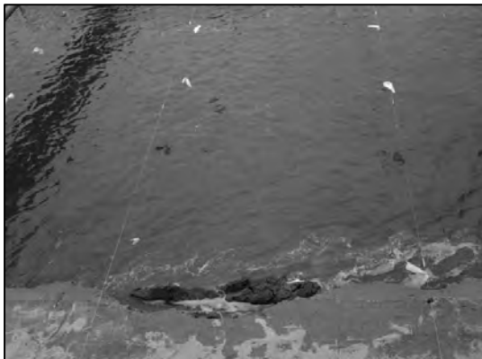
Figure A.39: Sliding of Bank
