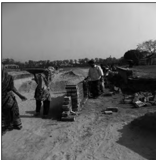
Figure A.9: Construction of Brick Wall
