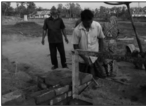
Figure A.19: Construction of D/S Tailgate
