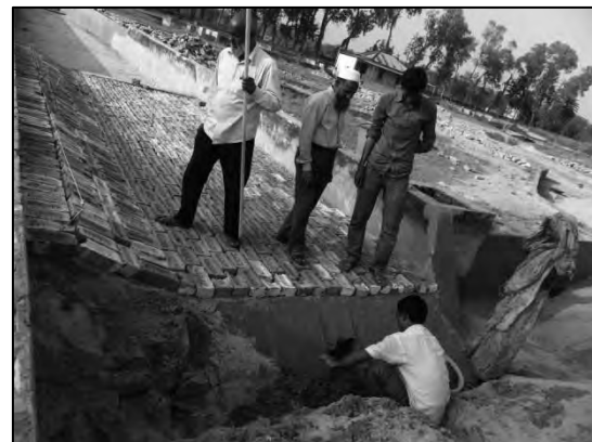
Figure A.14: Connecting the Backflow Pipe
