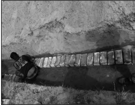
Figure A.5: Construction of Model Boundary
