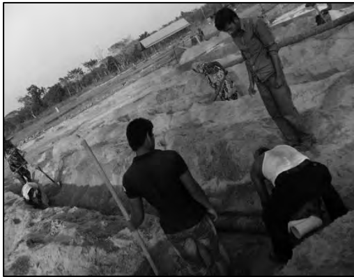
Figure A.13: Placing of Drainage Pipe
