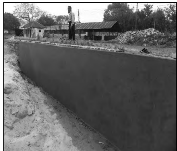
Figure A.10: Plastering Work at Boundary
