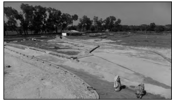
Figure A.20: Completion of a Boundary for Total Model (T-0 to T-20)
