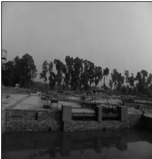
Figure A.27: Downstream Storage Pool
