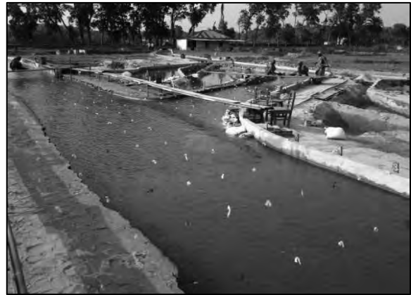
Figure A.38: Bank Erosion at Unprotected Condition
