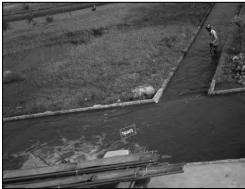
Figure A.31: Re-circulating Reservoir
