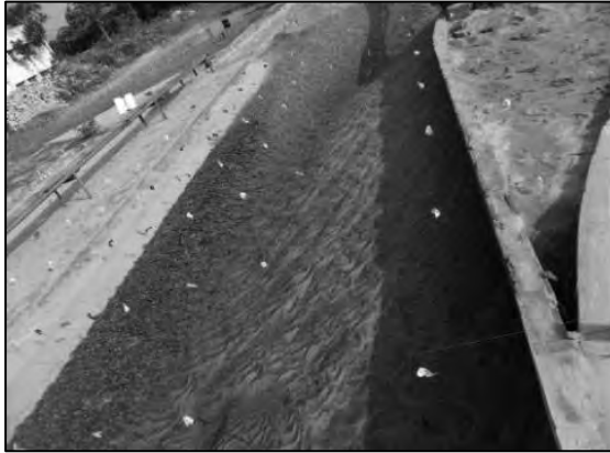
Figure A.47: Launching Behaviour of Geo-bag (738 kg)
