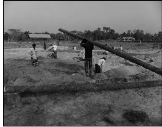
Figure A.12: Carrying the Drainage Pipe to the Position
