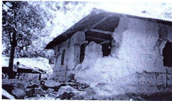
Figure 2.9: Failure of an earthen house due to July, 2003 Barkal Earthquake (Islam, 2002).
