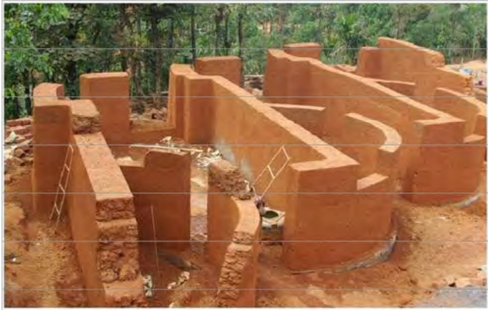
Figure 2.3: Rammed Earth Construction Underway in India (Source: www.banasure.com ).
