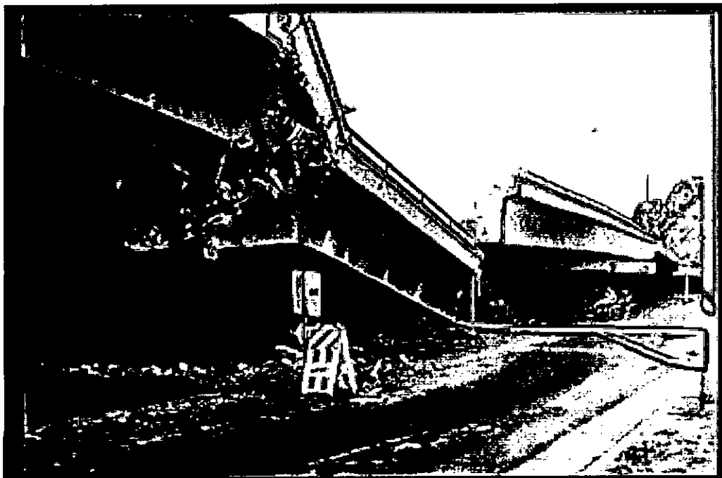
Fig 2.13 Superstructure Failure of a Flyover Bridge due to Earthquake (Kobe Earthquake)
