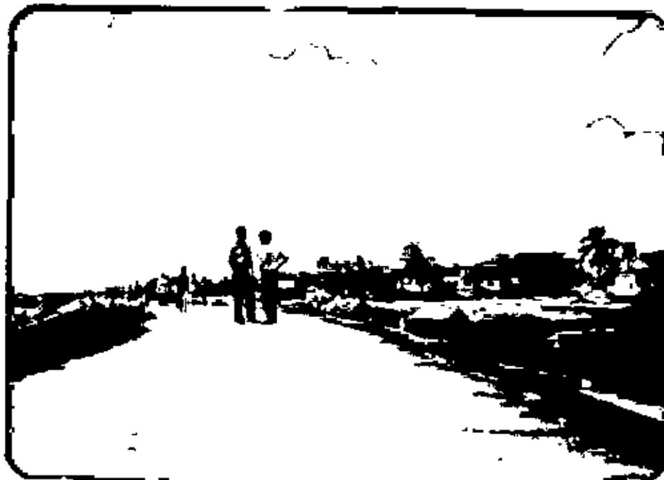
Embankment top levelled for use of pedestrians at Lalbagh area.
