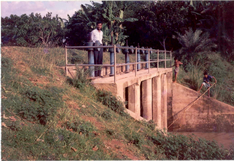
Photo 1: Suktajur Project: 5 vent regulator over Chuller Khal, view from river side,(Date : 16-8-94)
