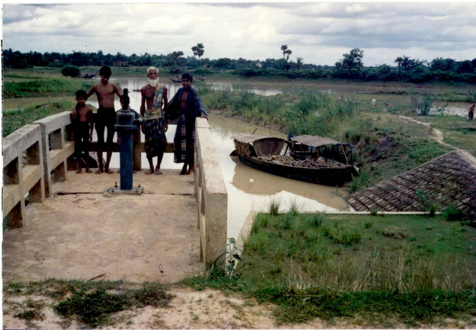
Photo 4: River side view of 1 vent Suktajuri Khal Regulator in good condition (Date : 16-8-94)
