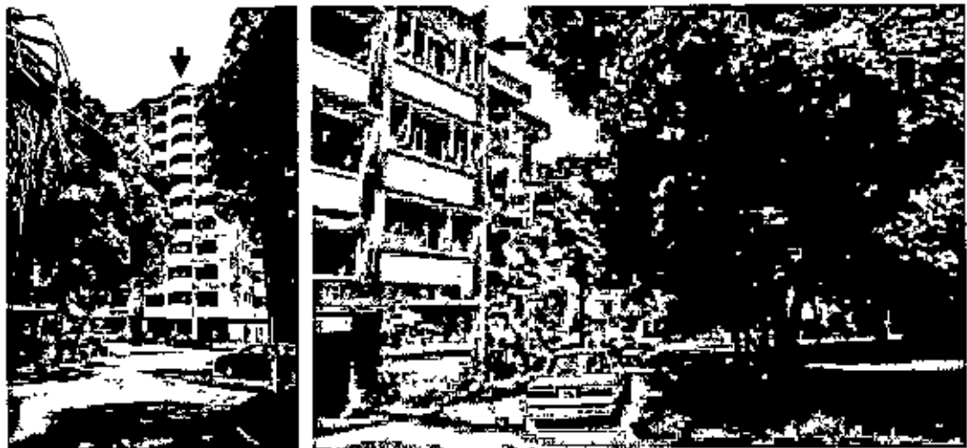
2.3a: Case study of 'Apartment with lift' 2.3b: Case study of 'Walk-up' type building
