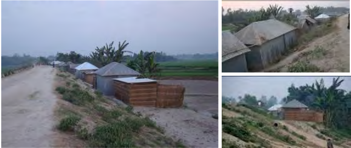
Figure 5.4: Settlement on the down-slope of the embankment.
