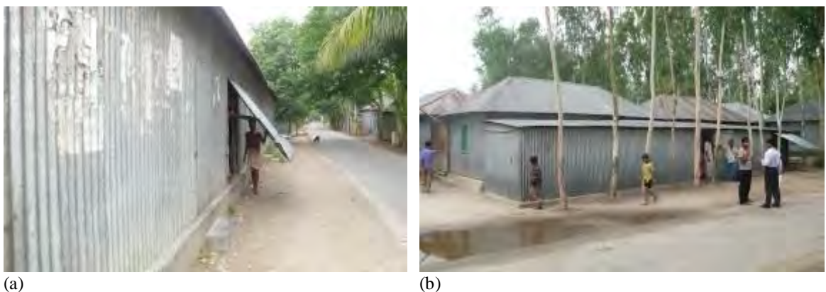
Figure 5.35 (a) and (b): The barren façade with shutter type opening of the HBE of sweet making and egg supply give a sense of the homestead with HBE includes it.
