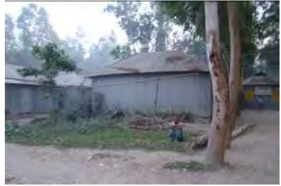
Figure 5.26: House of floating dwellers without proper plinth.
