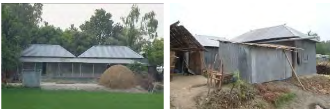
Figure 5.28: Use of C.I. sheets as a roofing material in permanent and floating homesteads.
