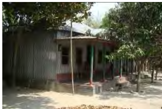
Figure 5.13: House with 'pucca' plinth.
