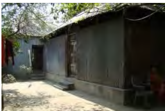
Figure 5.30: Use of C.I. sheets as an enclosing material.
