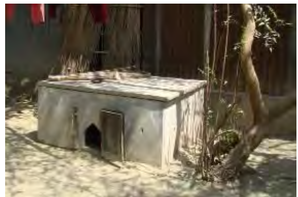
Figure 5.19: Concrete slabs are used to build the chicken shed.
