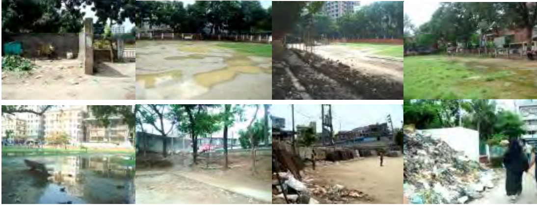
Figure 6.32: Physical condition of studied areas (planned & unplanned)
