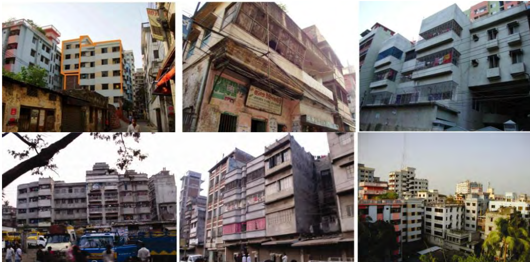
Figure 20: High dense building pattern in study area
