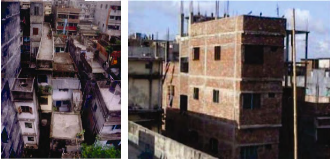
Figure 15: Poor condition of old Dhaka
