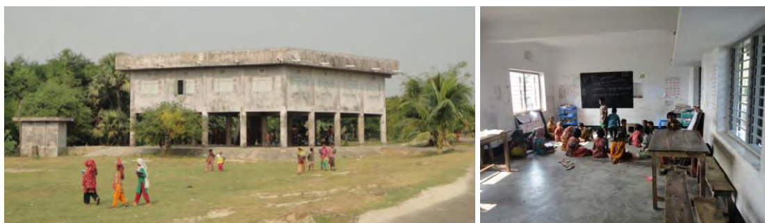
Fig 5.29: Cyclone shelter in Char Gangamati is used as educational institution in normal time.
