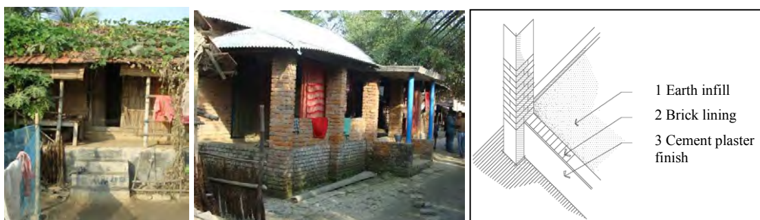
Fig 4.21: Construction of plinth with compact earth with brick lining is a popular practice in Maynapur.
