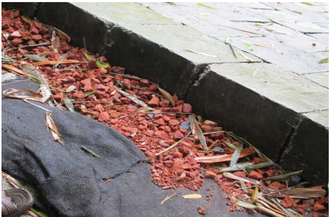
Figure 3.4 Brick chips used between concrete blocks and treated jute geotextiles
