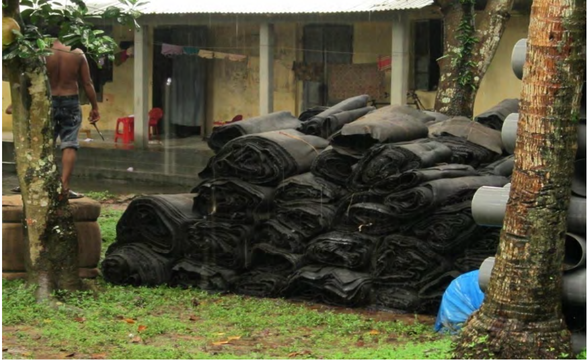
Figure 3.1 Treated JGTs that were used for river bank protection
