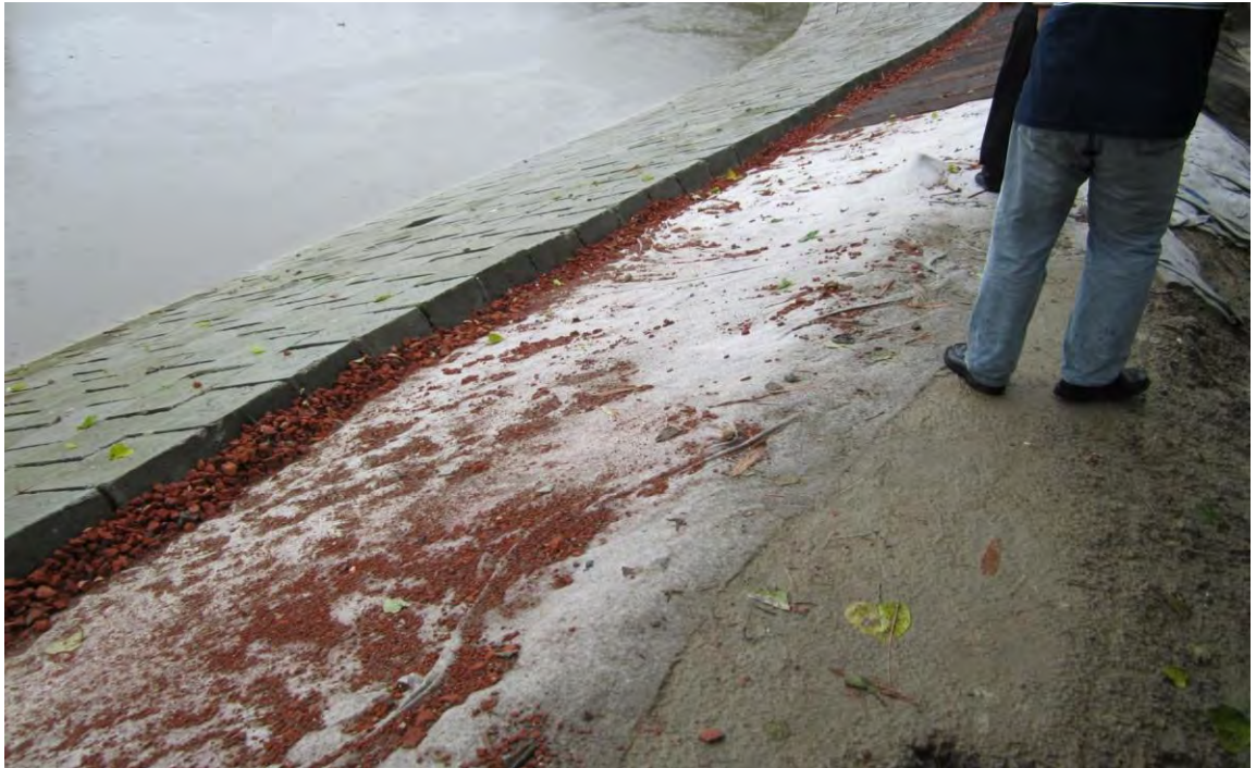
Figure 3.3 Synthetic geotextile used for river bank protection
