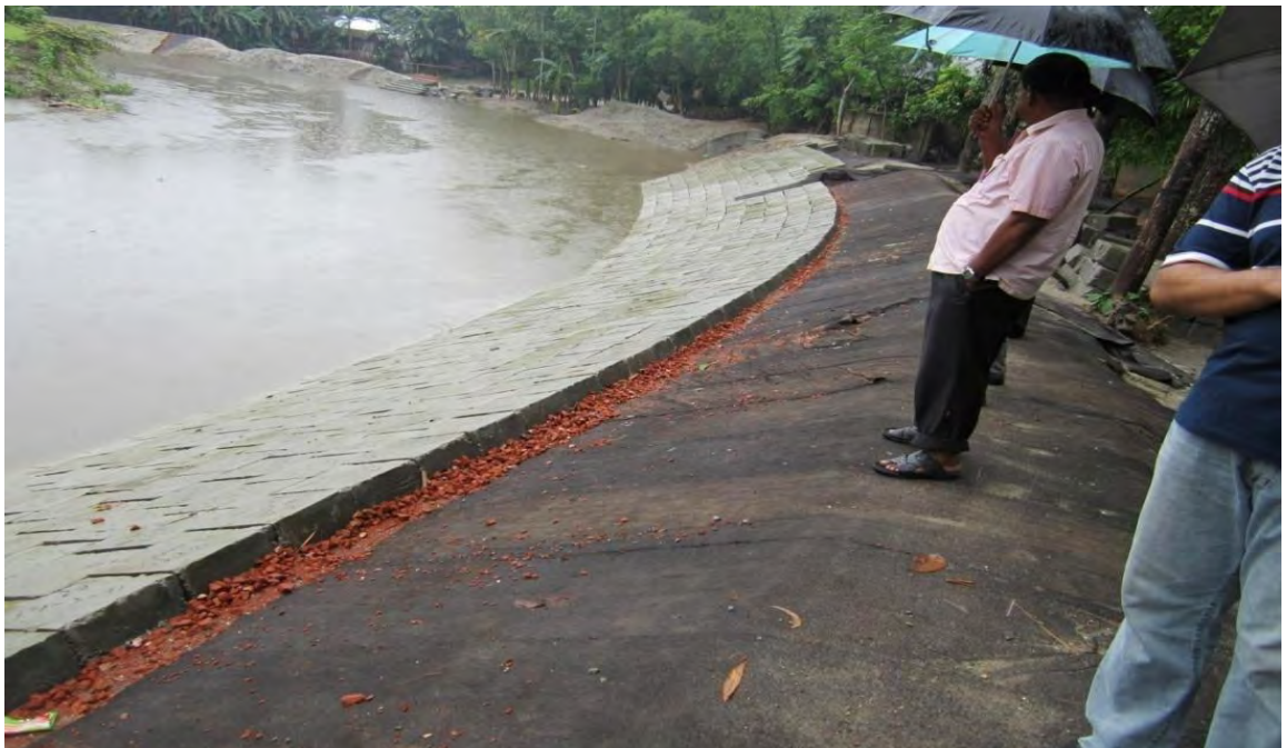
Figure 3.2 River bank protection using treated JGT
