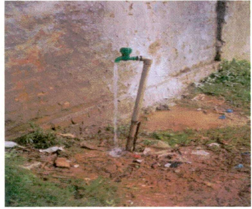
Figure 5.11: Wastage of huge amount of water due to high pressure (Boruda, Date: 23-11-02)
