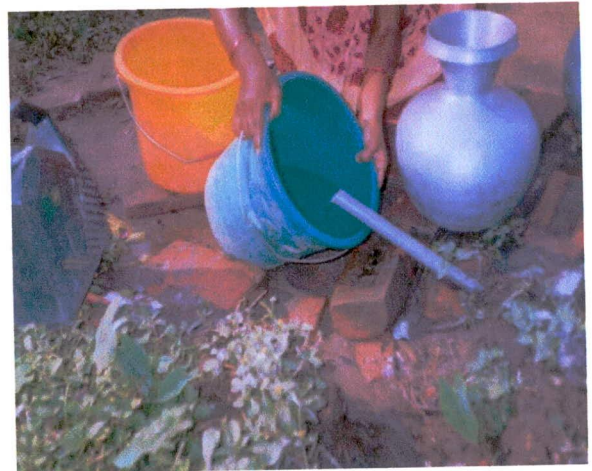
Low pressure at house connection (North Chayabithi, Date: 23-11-02)
