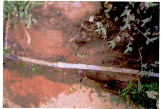
Leakage of pipeline (South Chayabithi, Date: 22-11-02)
