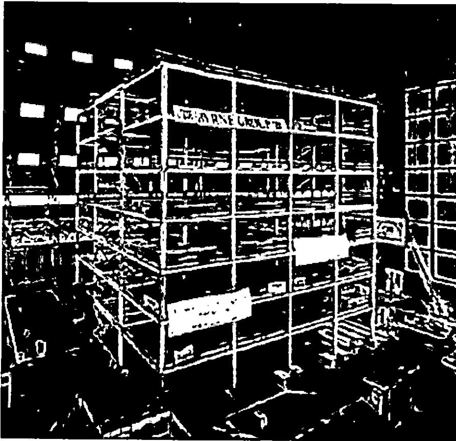
Figure 4.1: Cardington EPCB building
