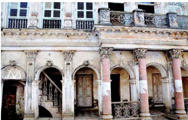
Fig-4.18: Partial View of Street Front Façade of Building no-3
