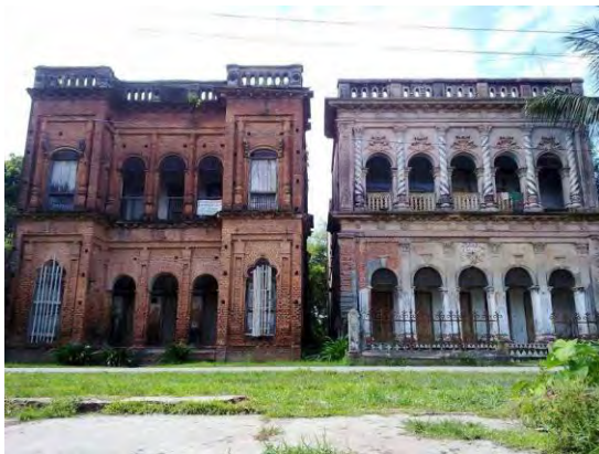
Fig-4.35: Street Front Façade of Building no-33 & 34
