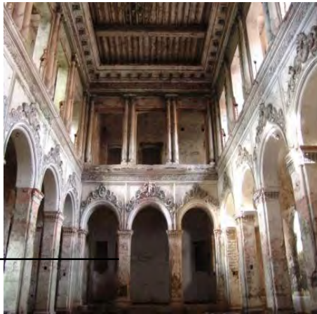
Fig-4.9 View of Double Heighted Hall Source: Field Survey, 2012
