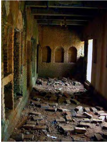
Fig-4.38: Front Room of a Consolidated Type Building
