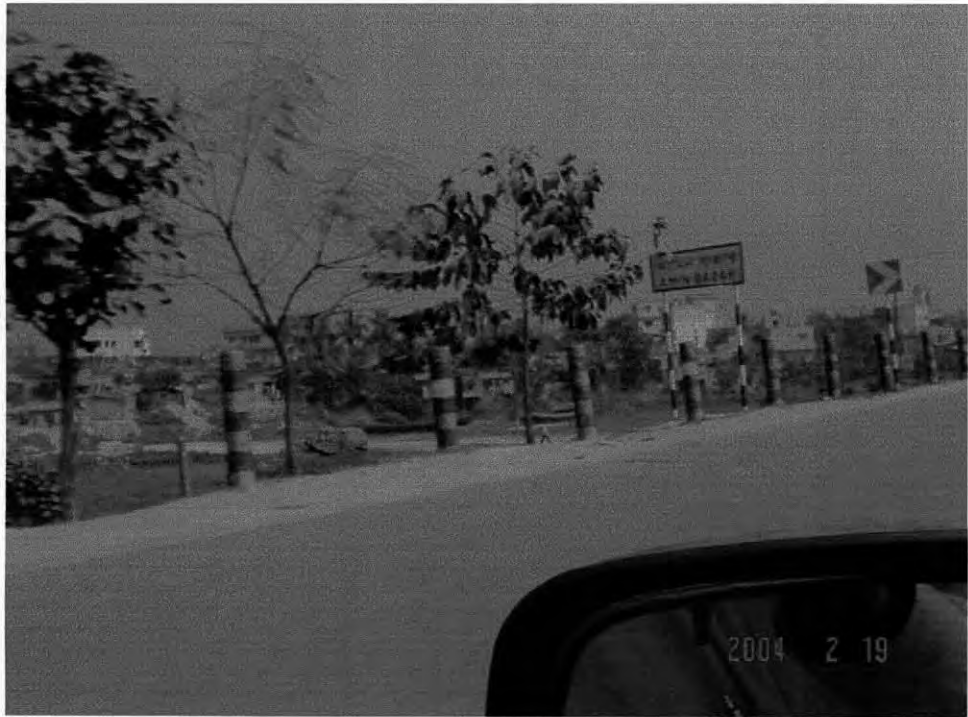
Figure 5.1 Sharp Bend Always Invites Hazard
