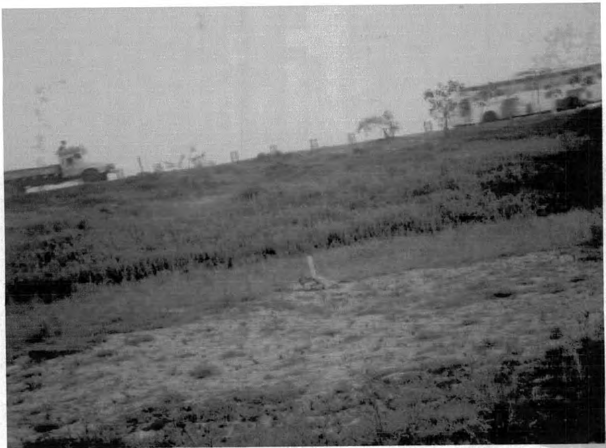
Figure B 4.2 High Embankment is a Unsafe Geometry by itself
