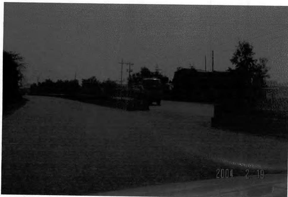
Figure 5.12 Frequent Opening at Median Invites right Angle Collision
