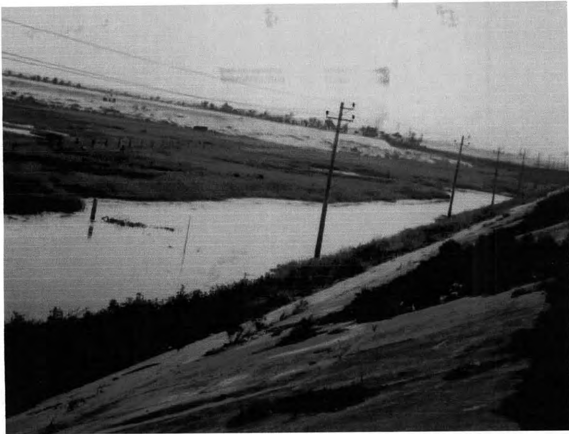
Figure B 4.3 Lack of Adequate Recovery Area is a Common Feature along this Corridor
