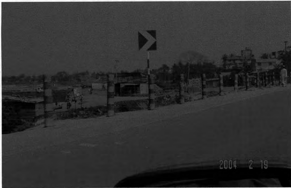
Figure 5.13 Chevron Should be Continuous
