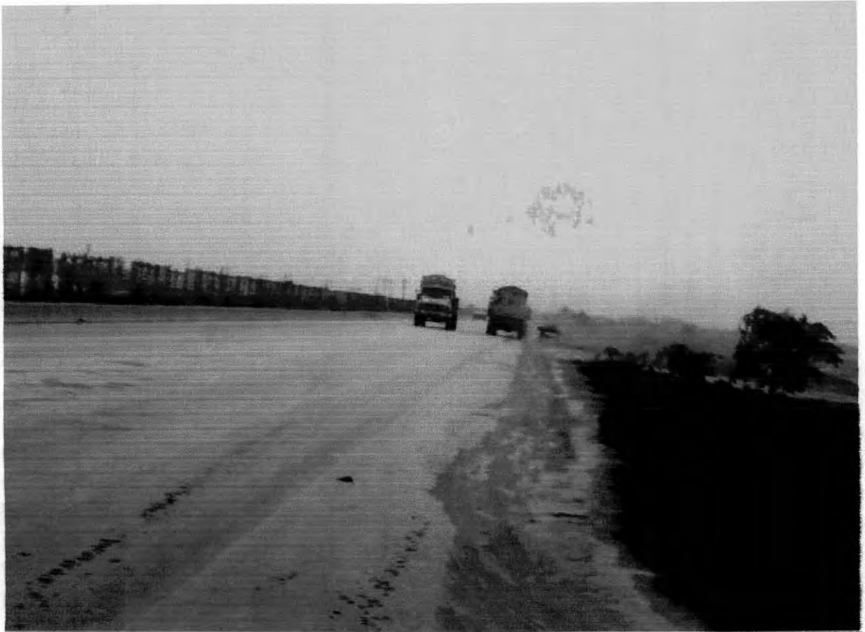
Figure B 4.13 Dangerous Contra Flow of Truck is a Common Scene in the Dual Carriageway Section of Dhaka-Aricha Highway, due to which Head on Collision still continues to occur.
