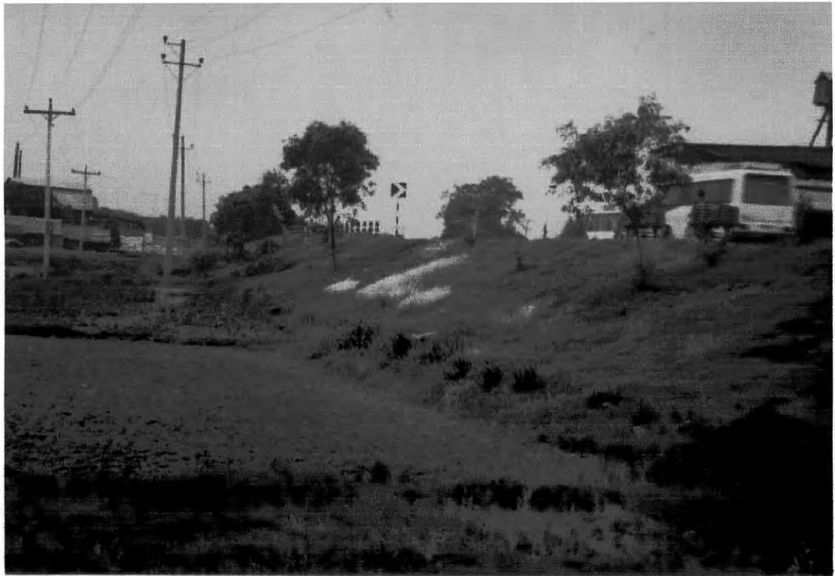
Figure B 4.9 Sharp Bend on High Embankment Further Aggravate the Risk of Overtum Accident
