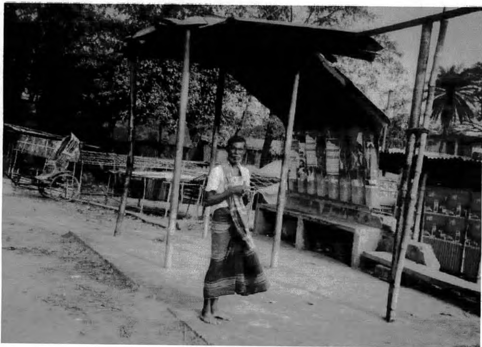
Figure 5.16 Newly Constructed bus shed at Baliha is Already Damaged
