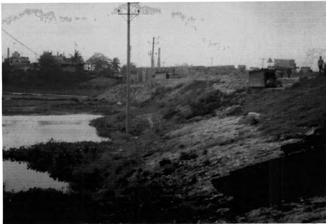
Figure B 4.4 Road Adjacent Areas Remain Fully or Partially Water logged Round the year
