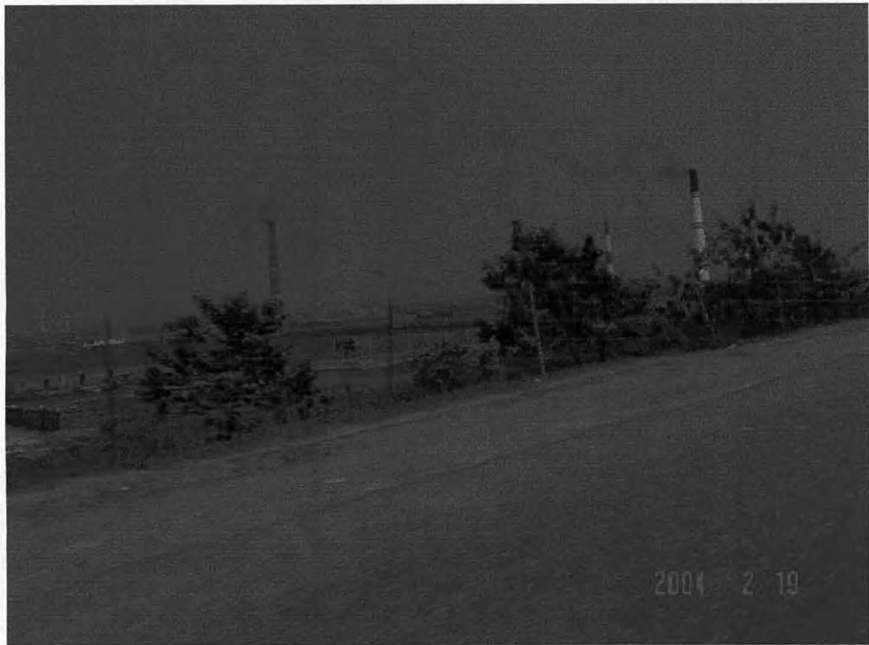
Figure 5.14 High Vertical Drop near Bridge is Hazardous
