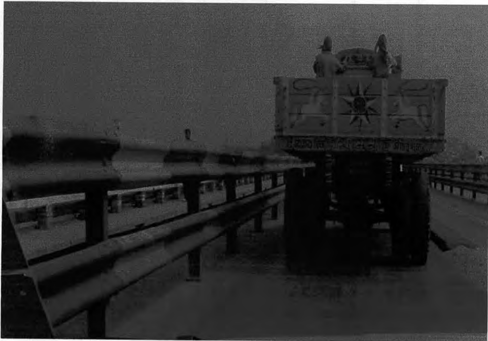
Figure 5.8 W-Beam Type Guard rail is an Ideal solution
