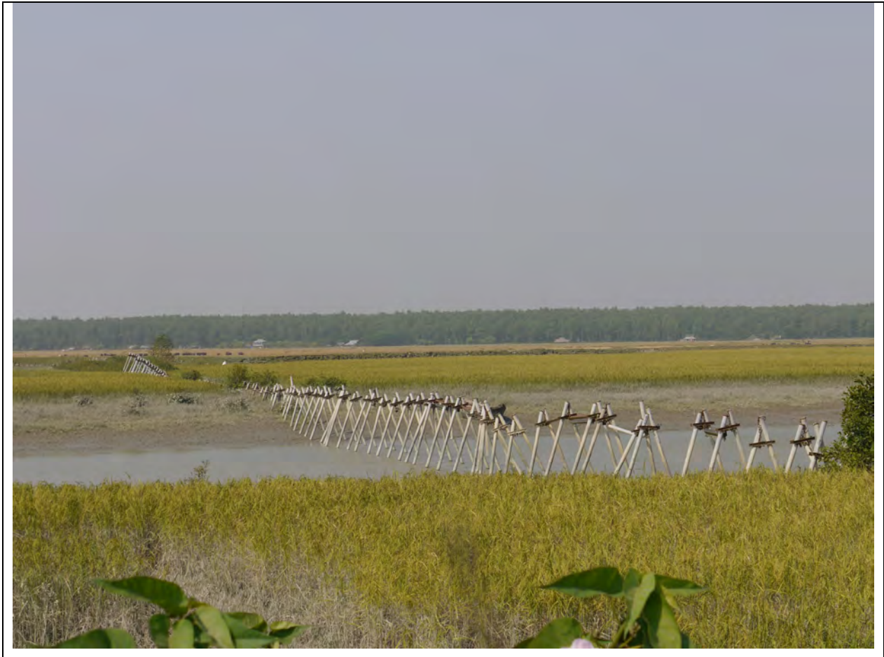
Figure 2.3: Permeable cross-dam constructed during MES-II on Bestin Channel in 1999.
