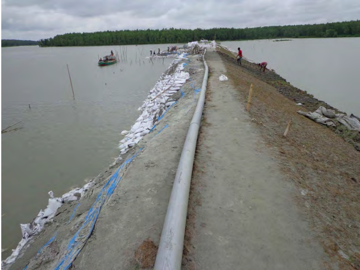
Figure-4.6: Closure over Montaz Channel (Looking towards Char Islam)
