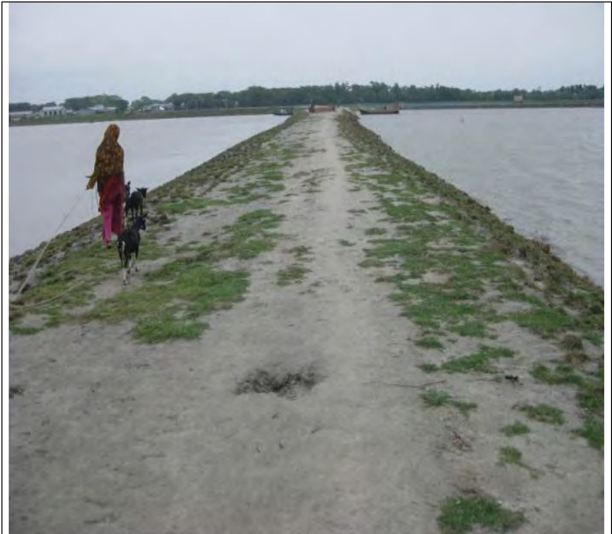
Figure 2.4: A solid cross-dam constructed during EDP on Bestin Channel in 2010.
