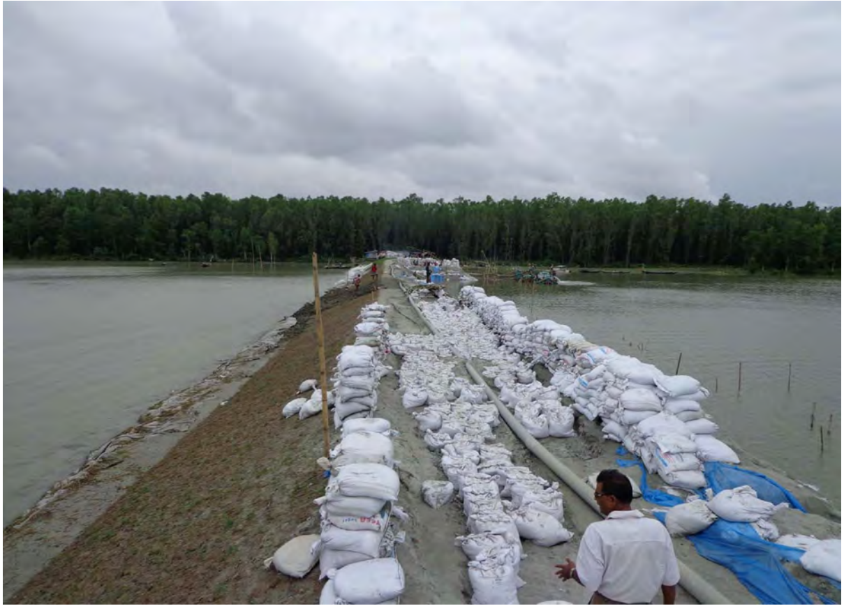
Figure-4.5: On-going closure over Montaz Channel (Looking towards Char Montaz)
