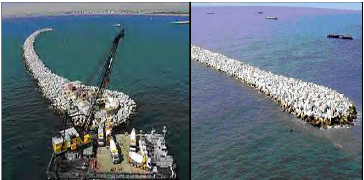
Figure 2.4(a): Large accropode units are placed by a crane and (b) after placing accropode blocks on offshore roundhead breakwater (Oman)
