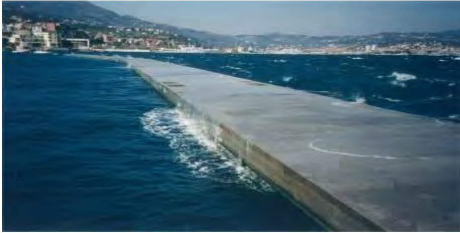
Figure 2.1: Box - floating breakwater (Fezzano, SP-Italy)
