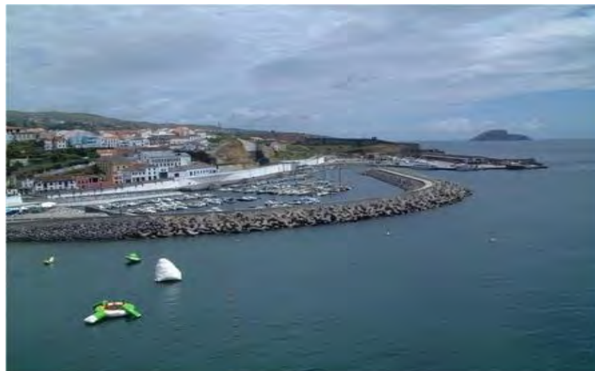
Figure 2.2: Emerged breakwater (Portland Harbor)
