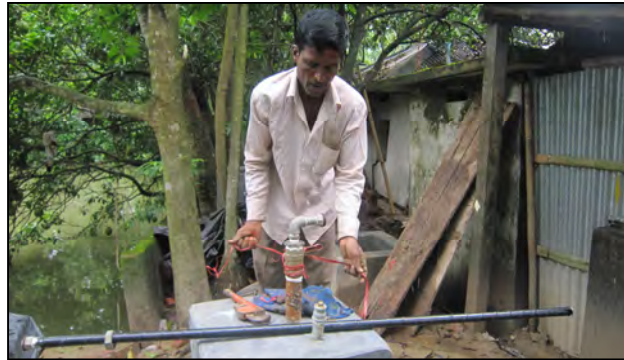
Picture 9.1: Opening of digester gate valve after one week.
