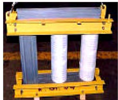
Figure 2.2: Transformer Core
