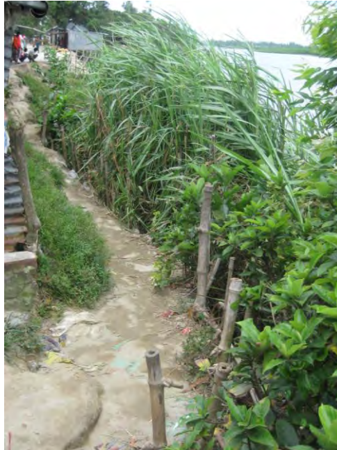
Figure 7.8: Planted nalkhagra to reduce hydraulic impact on the bankline at Randhunibari
