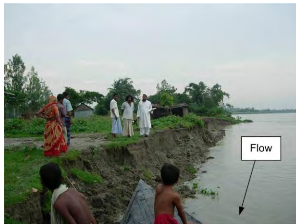
Figure 5.5: Erosion at the downstream bend of the study area (D)
