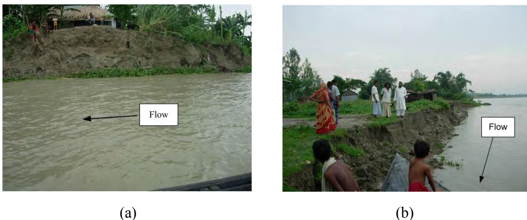
Figure 1.4: Erosion at Shuvogacha bend along the right bank of the Jamuna River
