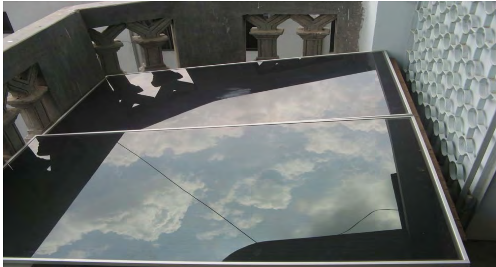
Figure 4.7: Two 50Wp thin film Solar panel [10]
