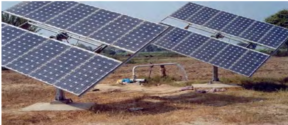
Figure 7.3: Solar water pumping with Solar Tracker [22].
